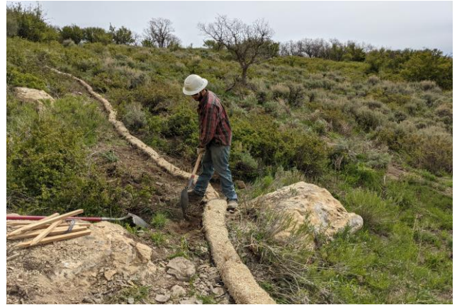
Installing Excelsior Wattle on the CC 697-08-53 Pad
