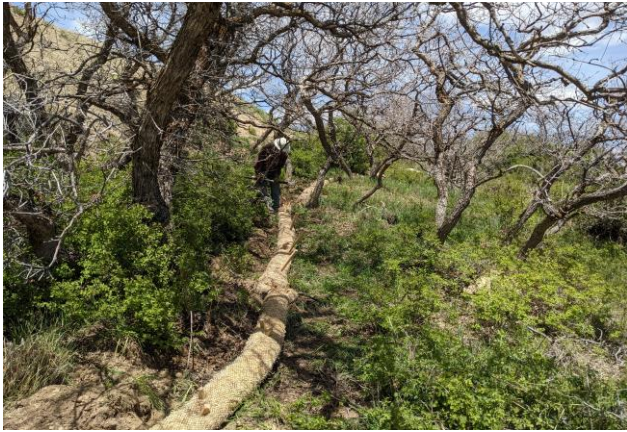
Excelsior Wattle Installed on East Side of Location
