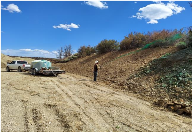
Applying Soil Amenities and Nutrients
