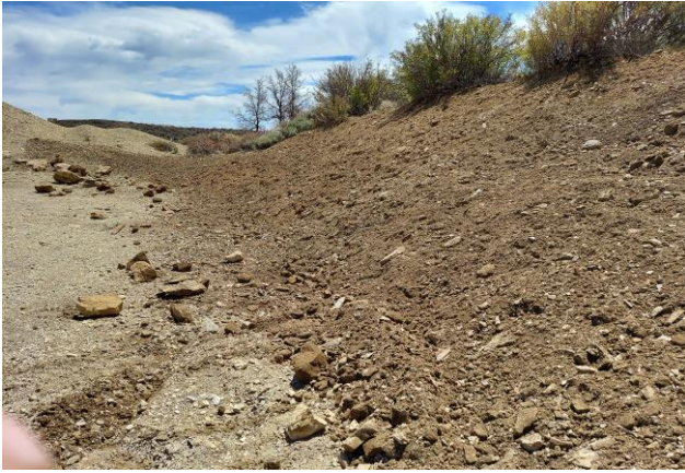
Material Pulled into the Cut Slope
