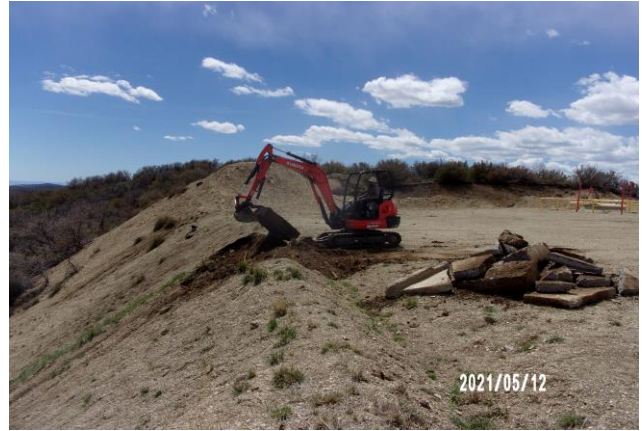
Pulling Concrete out of the Containment Berm
