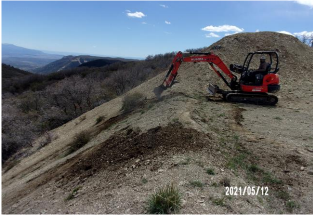
Pulling Concrete out of the Fill Slope
