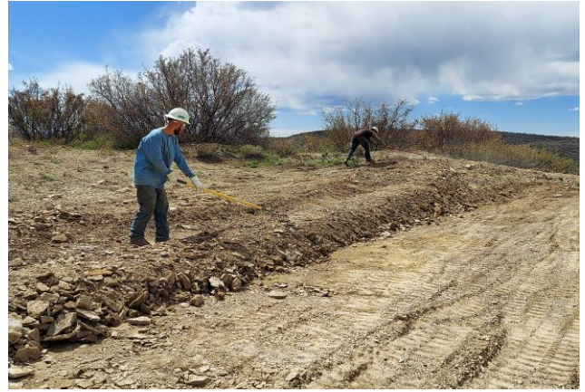
Hand Raking Seed to Incorporate into Soils
