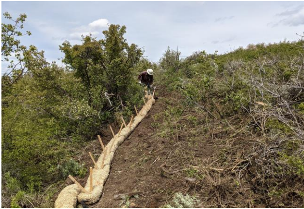
Installing Excelsior Wattle on the CC 697-08-53 Pad
