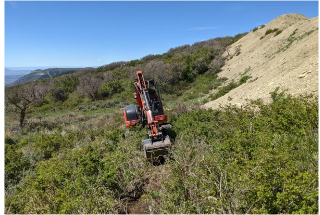
Removing Existing Vegetation to Install Excelsior Wattle
