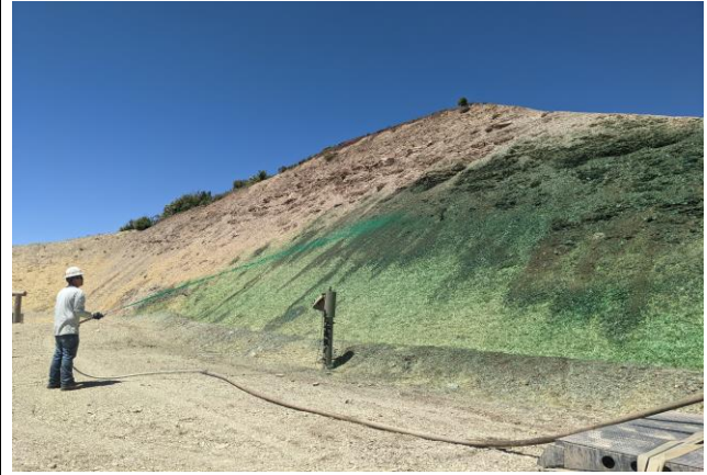
Applying Liquid Soil Amenities and Plant Nutrients
