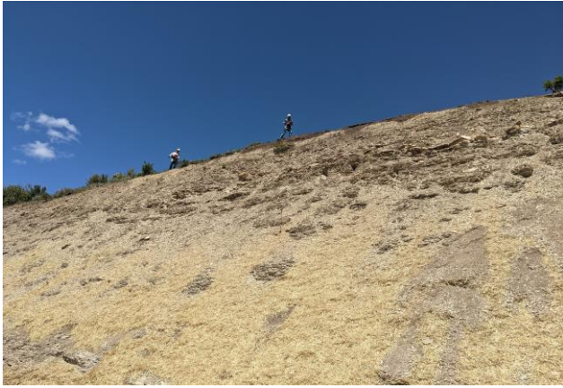
Broadcasting QuickGuard over CC 697-09-61 Cut-Slopes
