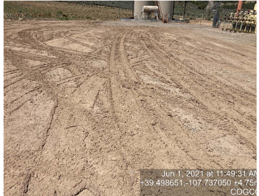
Lack of stabilization/compaction
