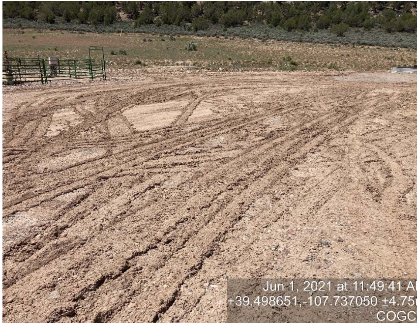
Lack of stabilization/compaction
