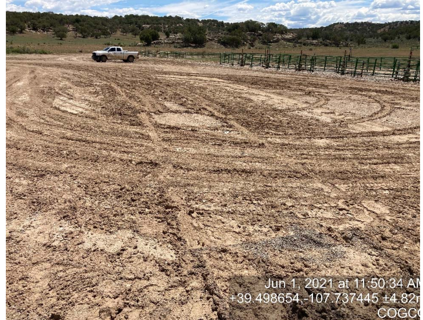
Lack of stabilization/compaction
