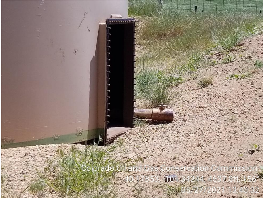
Photo 5 – Clean Out Plate STILL OFF – Wildlife Hazard
