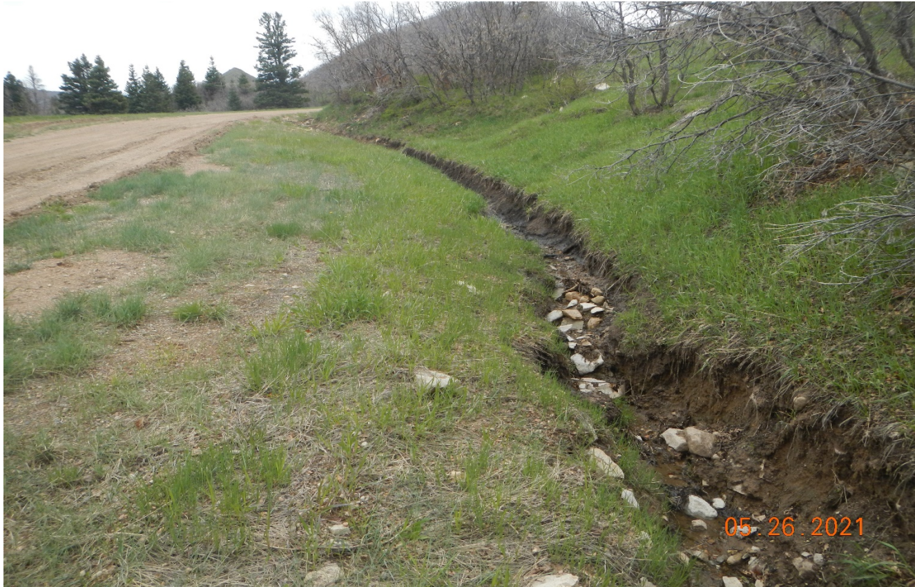
Photo 1. Facing southeast ascending the hill toward the location. There is erosion occurring along the road. BMP's are needed in this area along the road to prevent further erosion.
