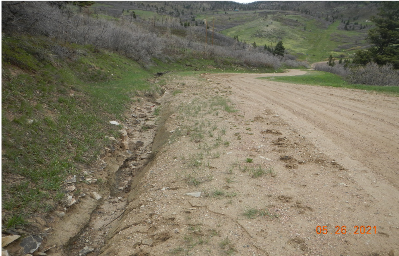
Photo 2. Facing northwest looking back down the road. There is erosion occurring along the road. BMP's are needed in this area along the road to prevent further erosion.
