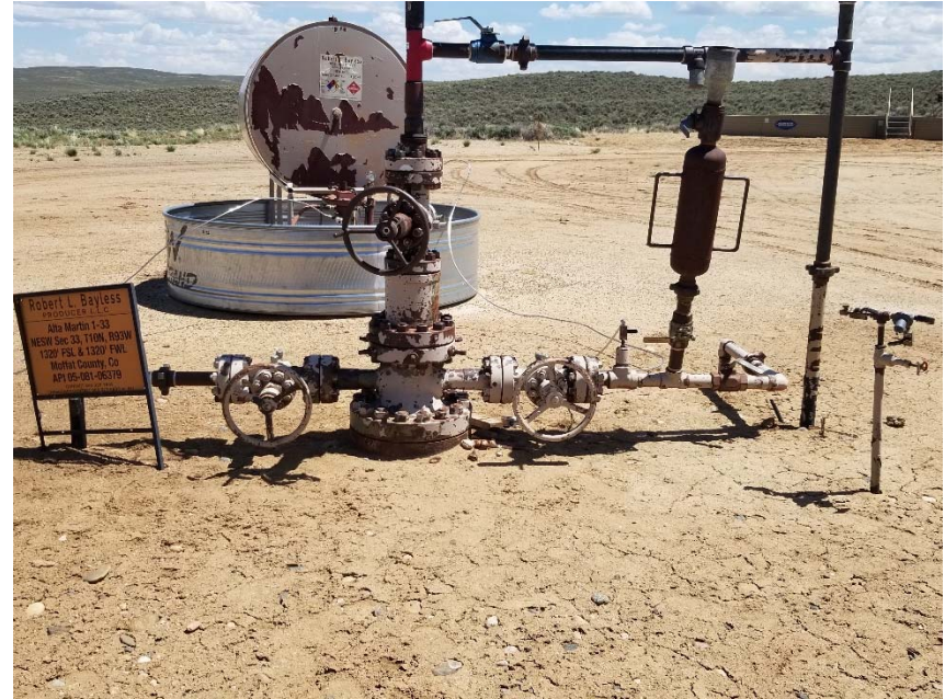
Photo 2. No bradenhead access apparent.
