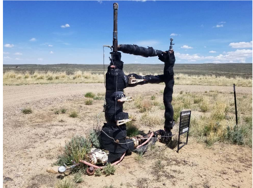
Photo 2. Hissing leak continues at wellhead.
