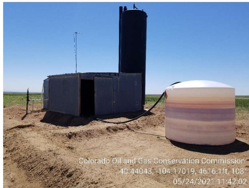
Photo 8 – Heater Treater and 40 BBL Produced Water Tank
