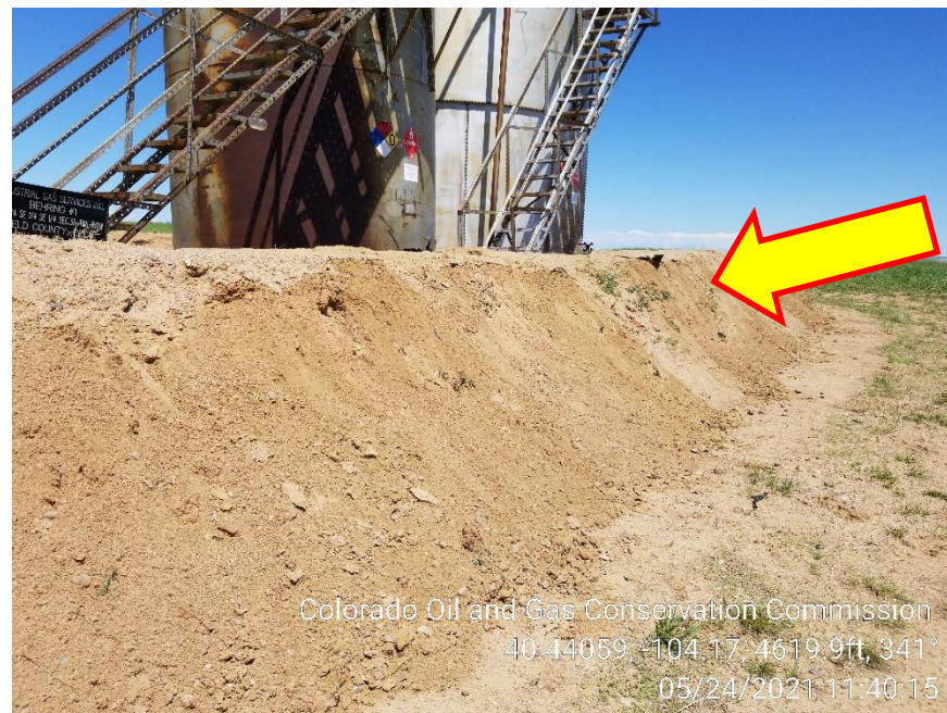
Photo 6 – Berm at Tank Battery have been resolved.
