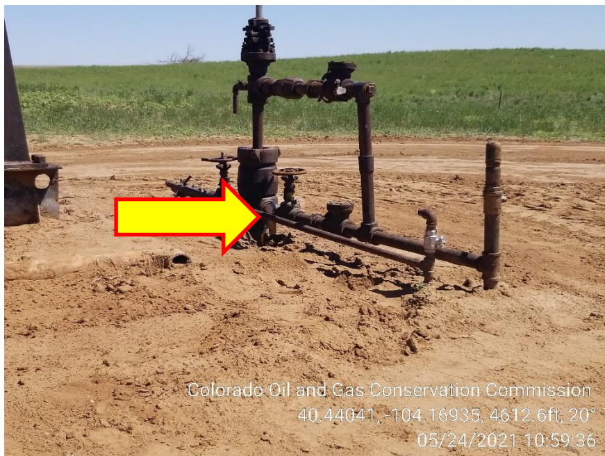
Photo 3 – Bradenhead has NOW been plumbed to surface
