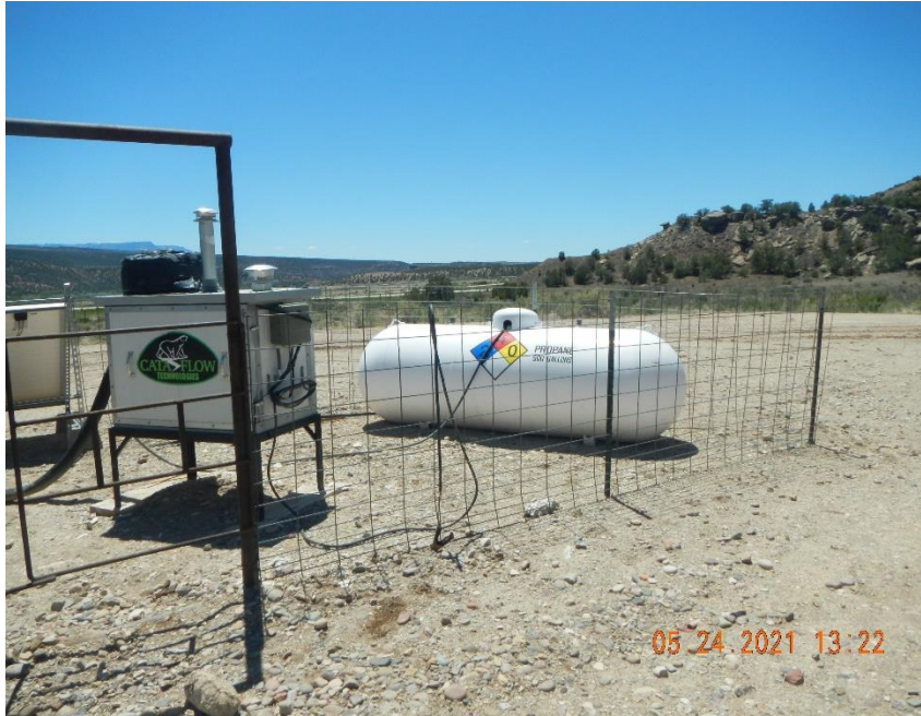
Propane LPG tank at well. CATAFLOW line heater at well.
