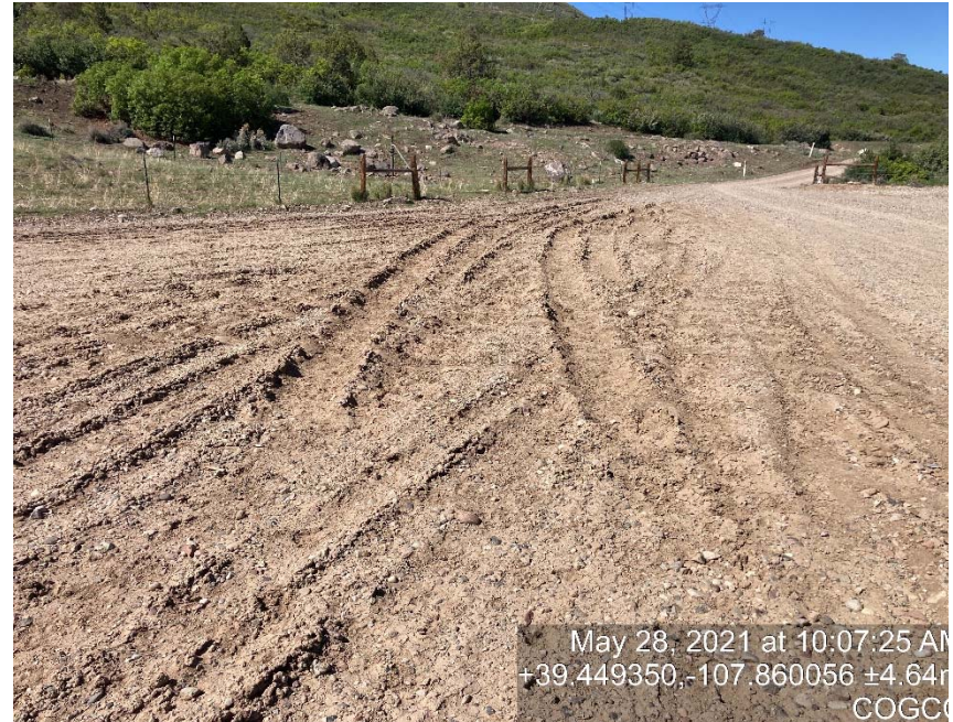
Lack of stabilization/compaction
