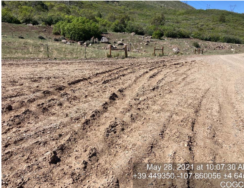
Lack of stabilization/compaction
