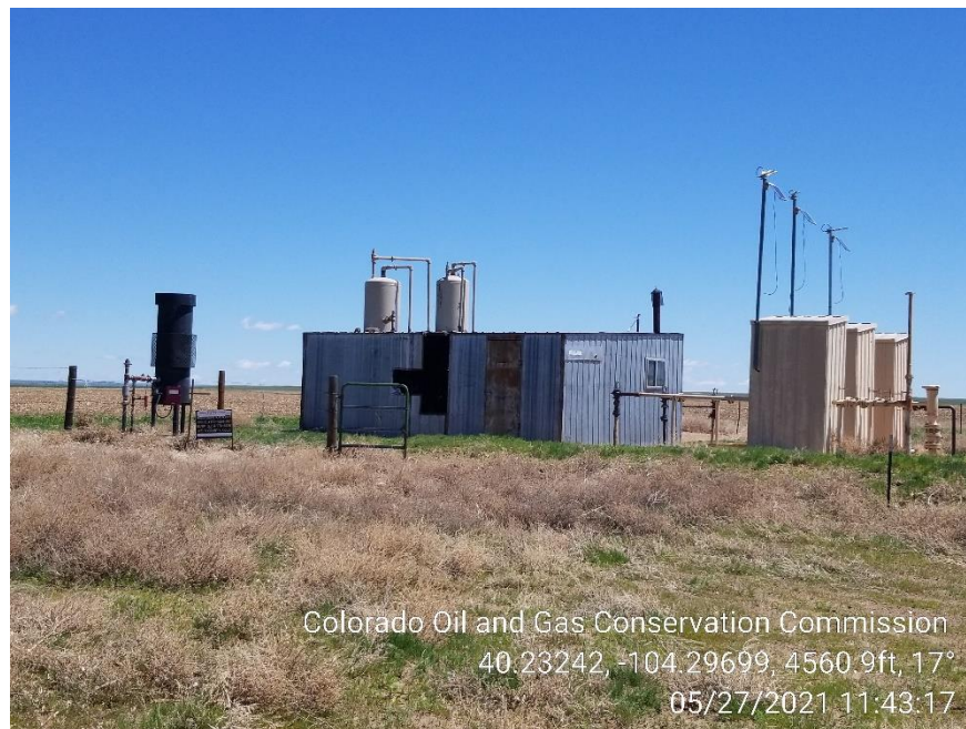
Photo 6 – Separators, ECD and Gas Meters – Weeds
