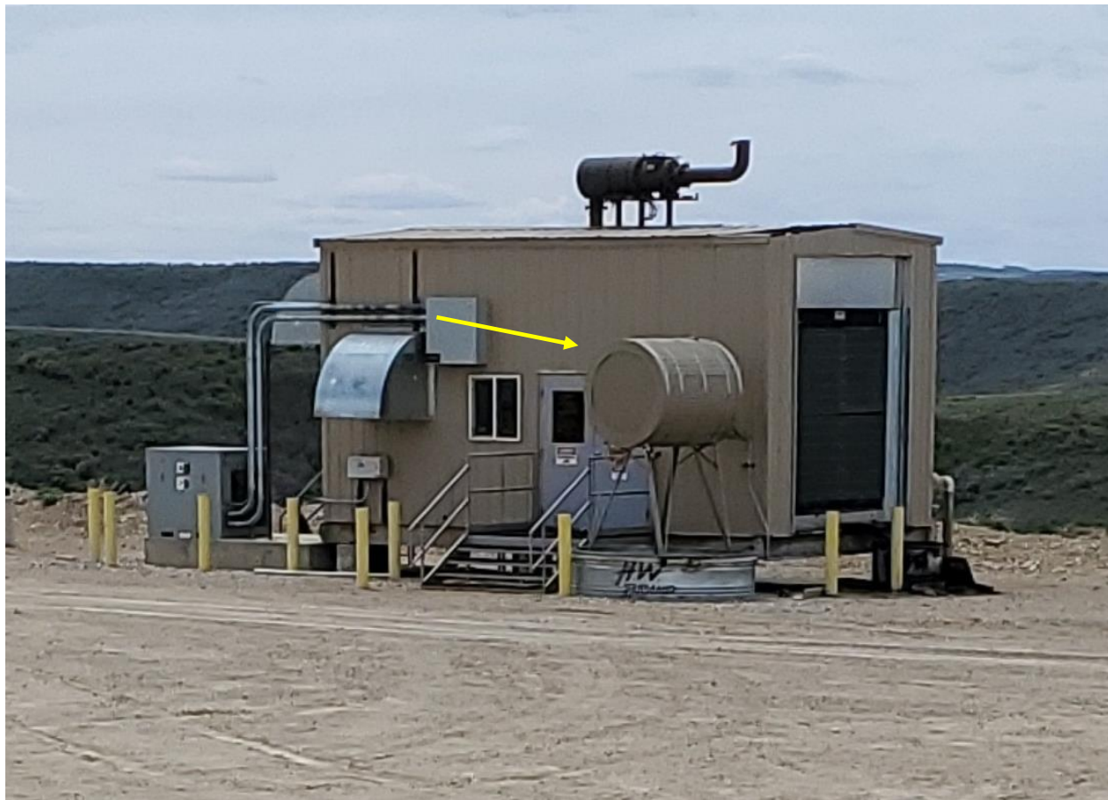
Photo 16: Photo shows tank in front of generator housing; sign or label not posted, or installed in a place where not visible.
