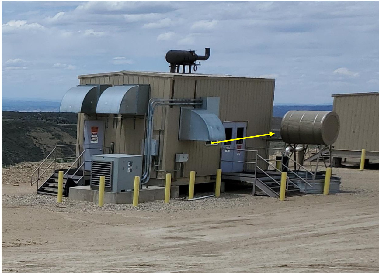
Photo 15: Photo shows tank in front of generator housing; sign or label not posted, or installed in a place where not visible.
