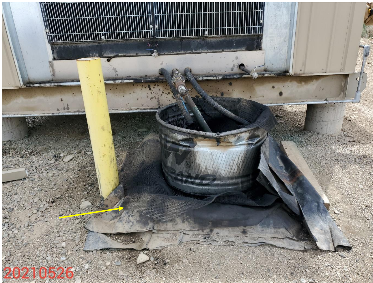
Photo 13: Photo taken from the north side of the generator housing. Photo shows tank installed to collect various chemicals from the housing unit. Photo also shows the containment BMP at base of tank; containment BMP is insufficient to prevent and/or contain a spill from the tank.
