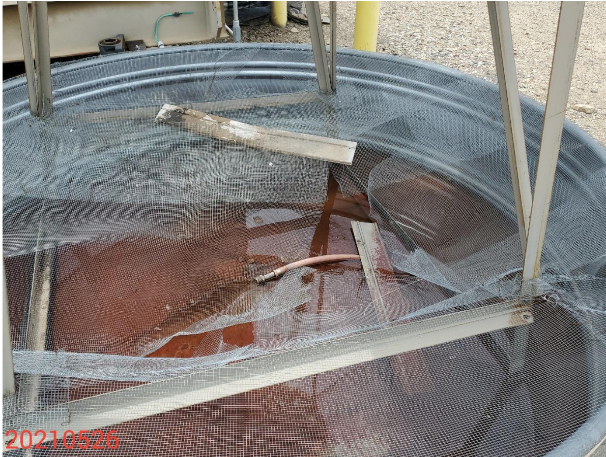
Photo 17: Continued from photo 16. Photo shows wildlife protection screen is not in proper functioning condition. Photo also shows various trash debris within tank.
