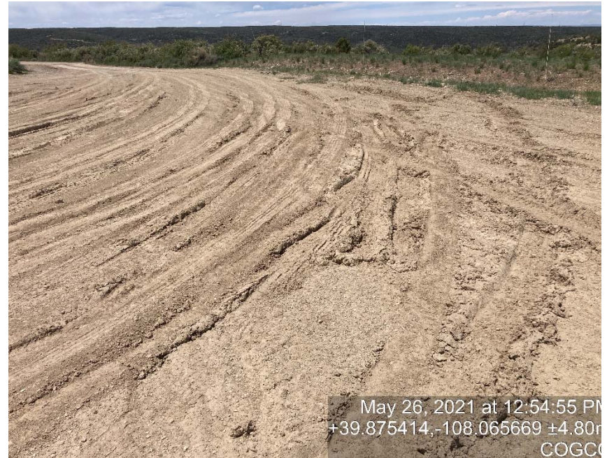
Lack of stabilization/compaction
