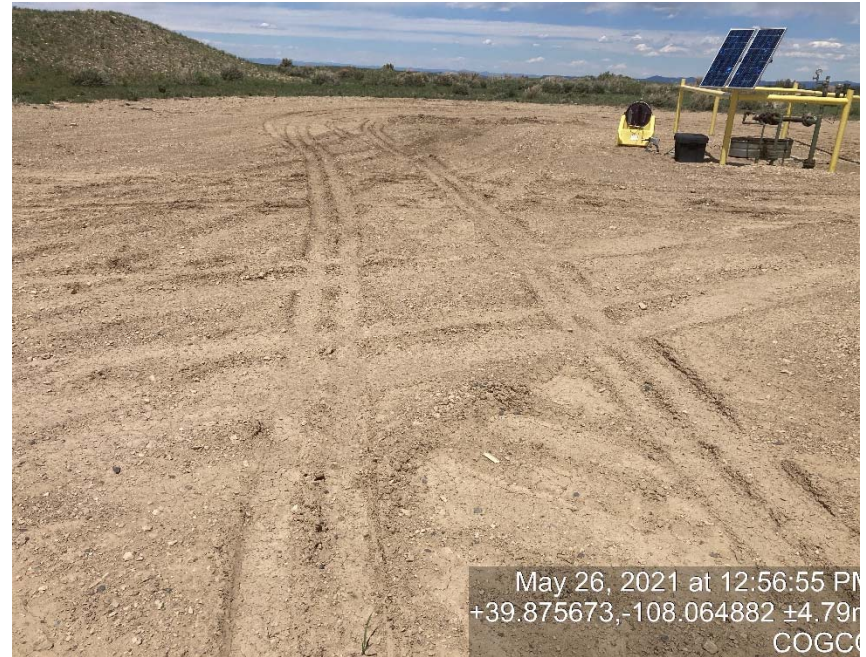
Lack of stabilization/compaction
