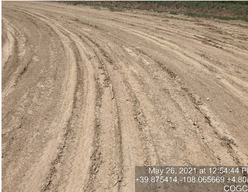
Lack of stabilization/compaction
