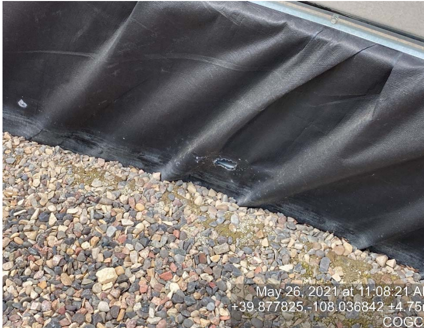
Hole in battery containment
