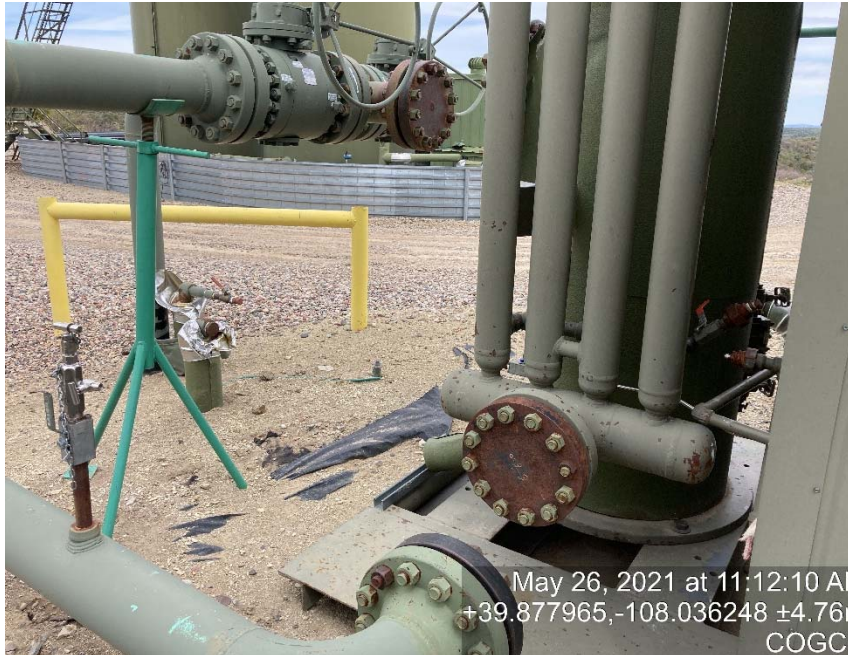
Dehy is disconnected (unused equipment)
