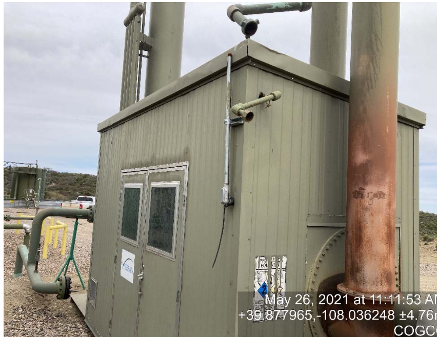
Dehy is disconnected (unused equipment)
