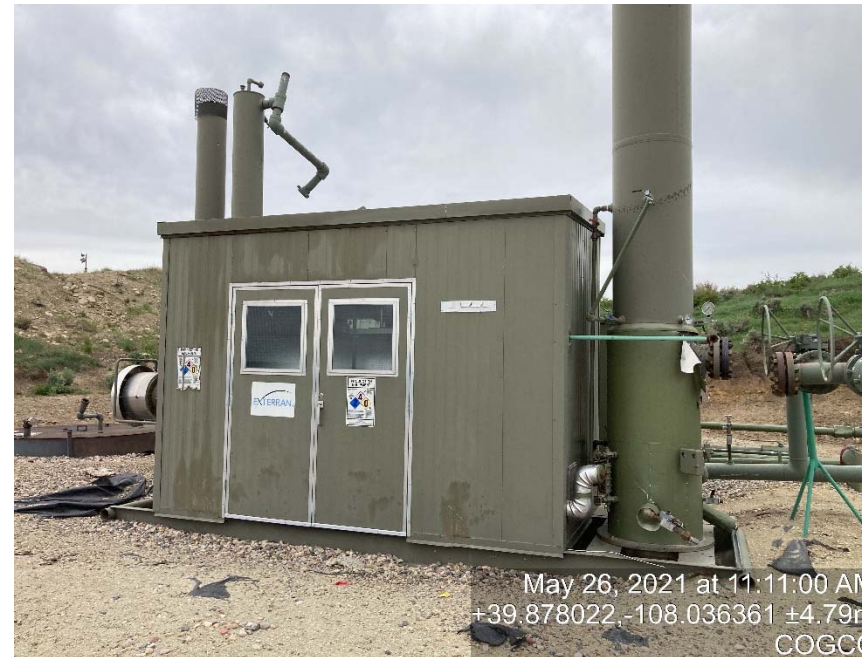
Dehy is disconnected (unused equipment)
