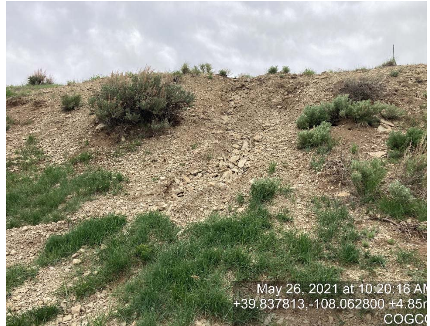
Erosion on fill slope
