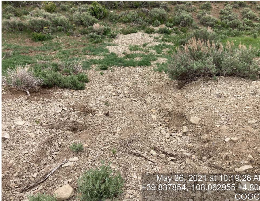
Erosion on fill slope
