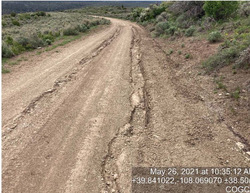
Lack of stabilization/compaction
