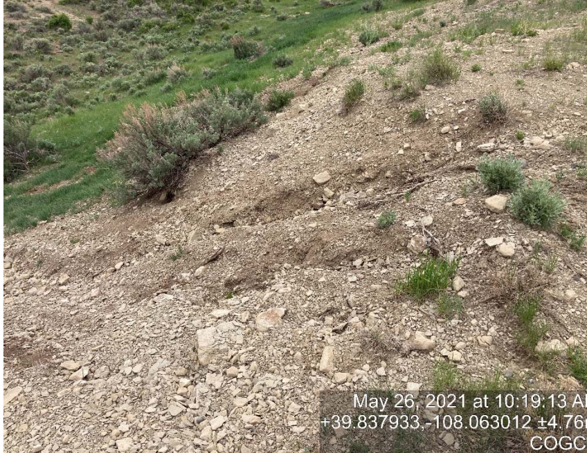
Erosion on fill slope
