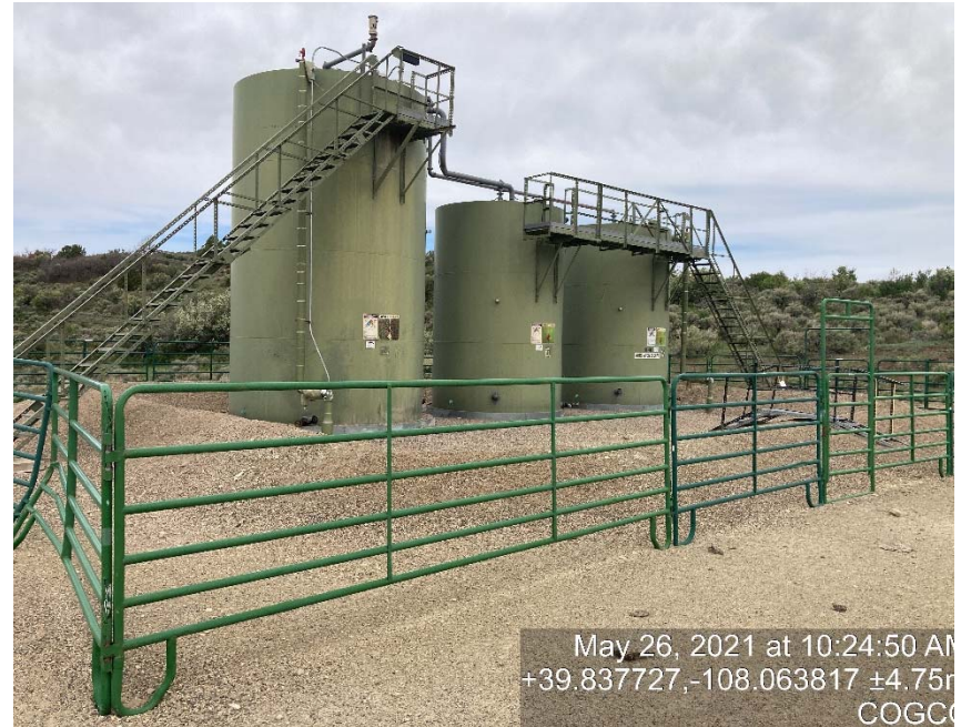
location/lack of battery signage
