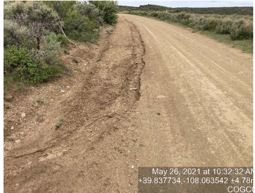
Lack of stabilization/compaction
