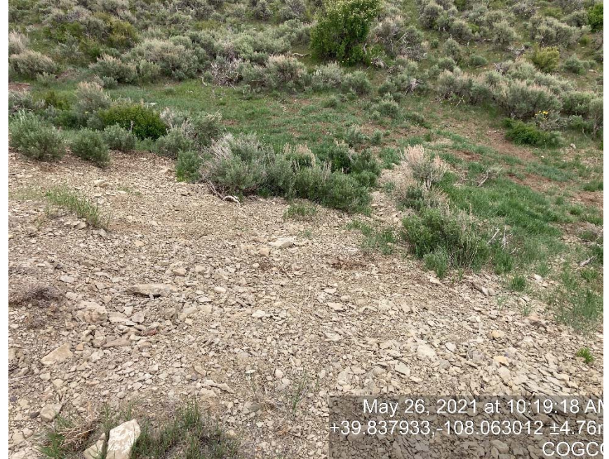
Erosion on fill slope
