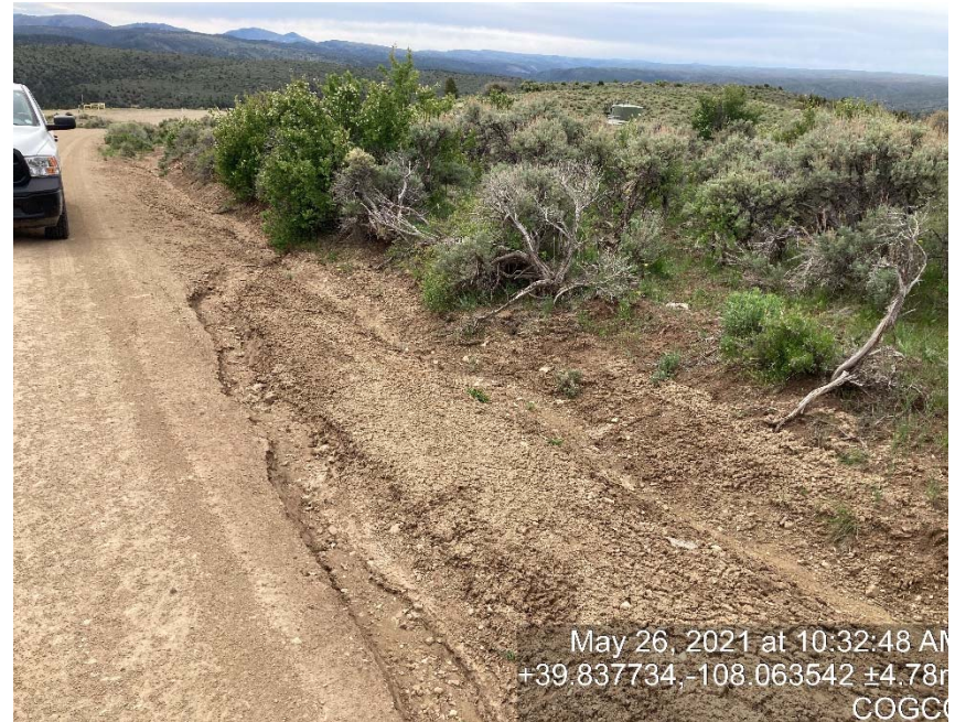
Lack of stabilization/compaction
