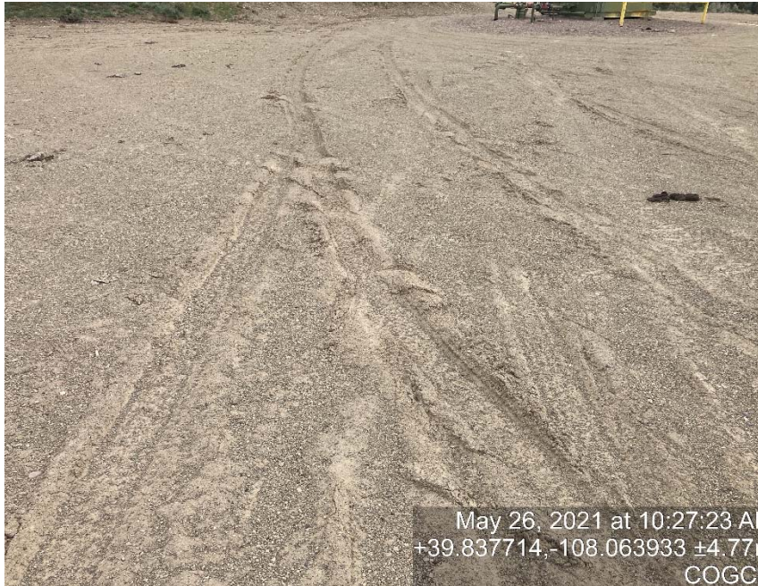
Lack of stabilization/compaction
