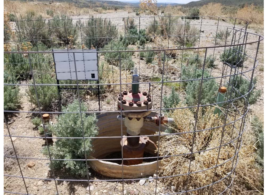
Photo 2. No bradenhead access apparent.
