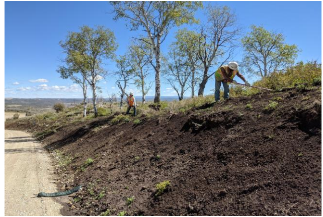
Hand Raking New Seeding along CC 697-03-07 Access Road
