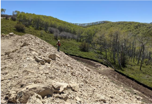
Broadcasting Temporary Seed over Rocky Fill Slopes
