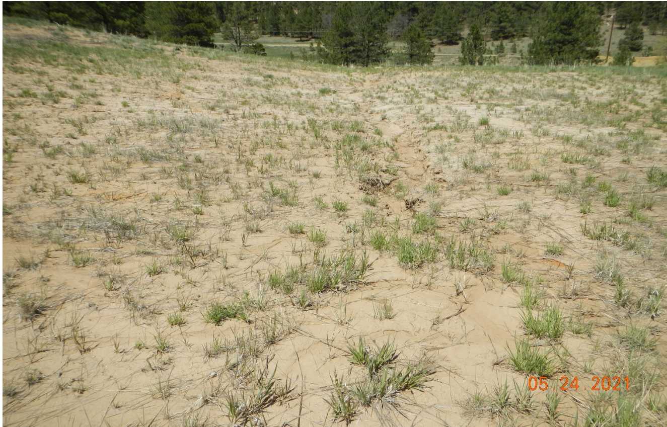
Photo 5. Facing north at the location. There is an erosion channel down the center of the location.
