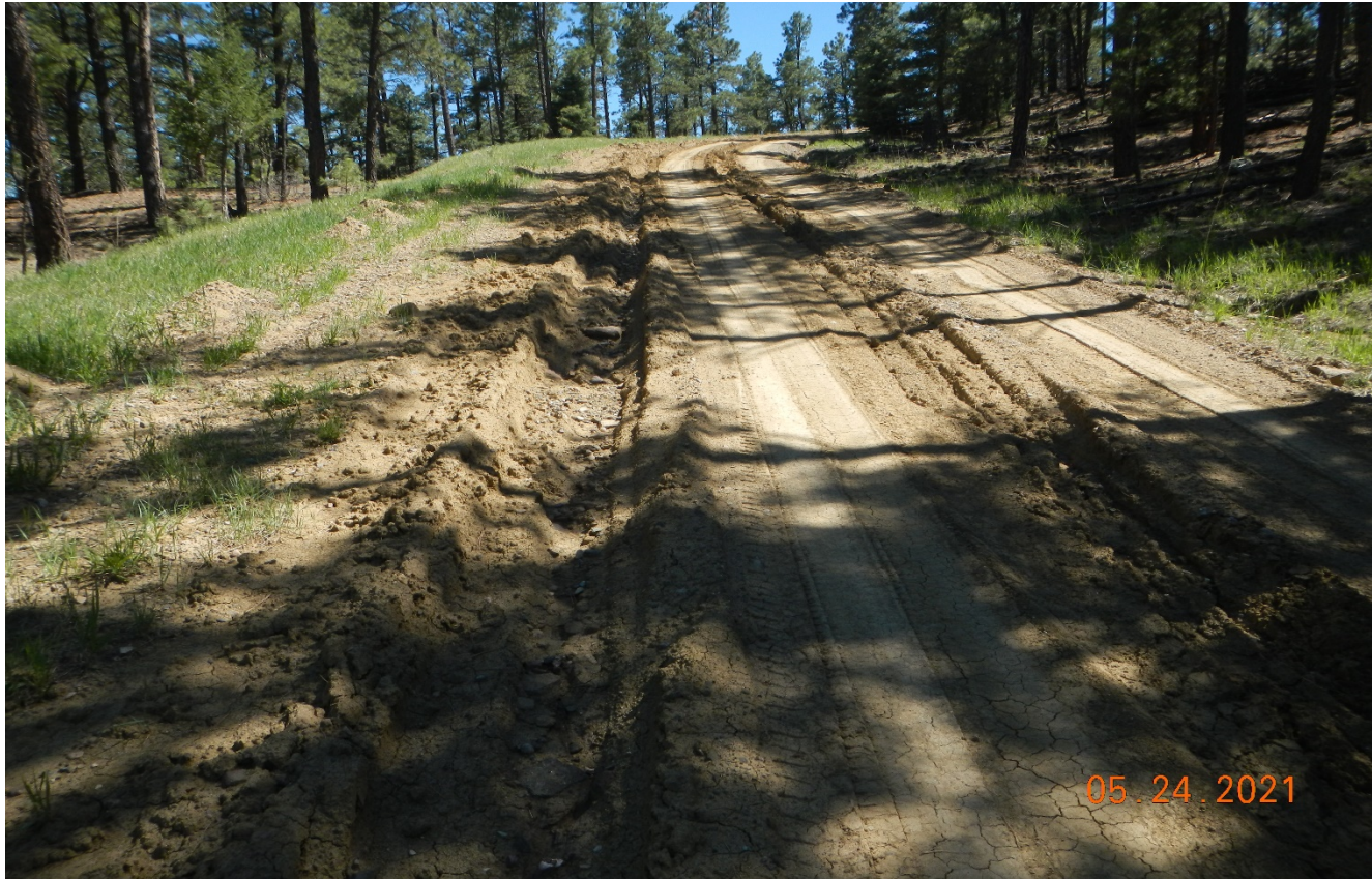
Photo 2. Facing southwest along the access road. There are areas along the road that have vehicle rutting and erosion.
