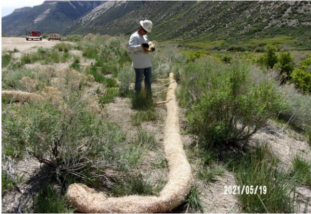
Installing Excelsior Wattle on CC 629-31-11 Pad
