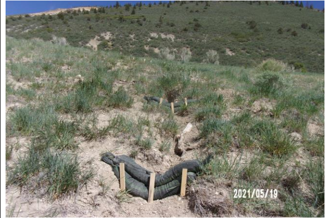
Erosion Channel Checked Up on CC 629-31-11
