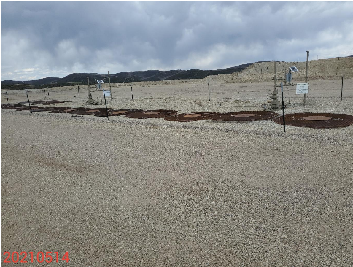
Photo 5: Photo taken from the wells. Permits for undrilled wells on the Location have been deleted. Photo shows conductor settings/cellars require closure and reclamation in accordance with Rule 406.e.
