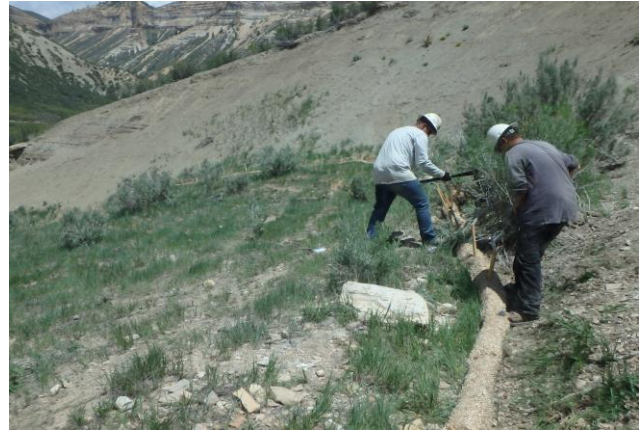
Installing Wattle on CC 629-02 Pad
