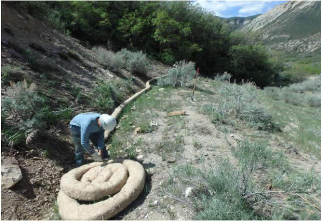
Installing Wattle on CC 629-02 Pad
