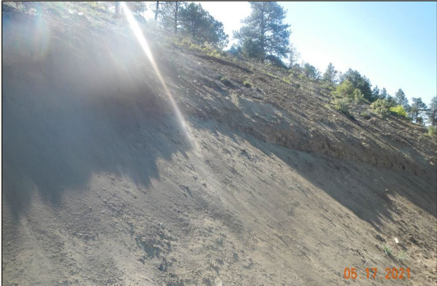
Photo 5. View of bare soils on the upper cut-slope and diversion. Long term soil stabilization measures need to be installed to stabilize soils here.
