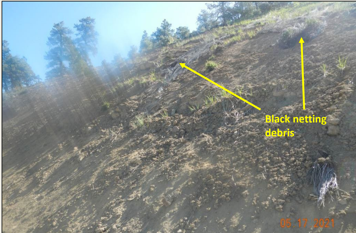
Photo 4. View of the upper portion of the eastern cut-slope. Revegetation remains sparse here. Black plastic netting debris needs to be removed.
