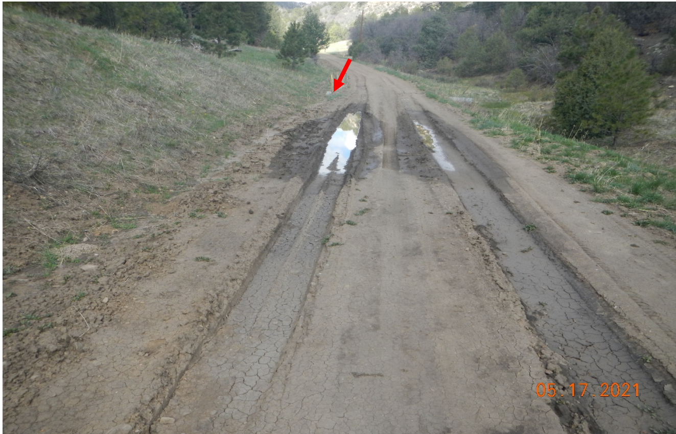
Photo 5. Stormwater is not directed toward the culvert (at red arrow) causing stormwater to accumulate on the road. Areas of rutting need to be stabilized. Previous corrective action was not performed
