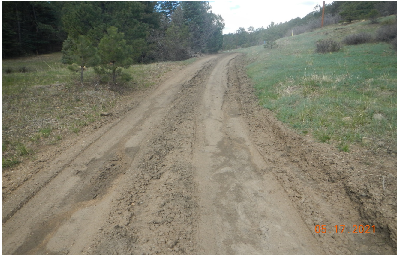
Photo 1. Facing southwest along the main road. There is vehicle rutting along the main road. Areas of rutting need to be stabilized. Previous corrective action was not performed.
