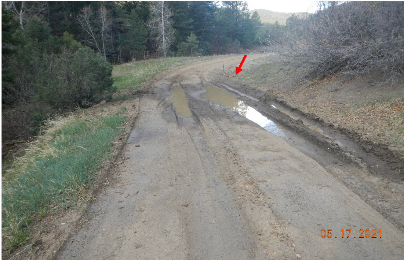
Photo 2. Stormwater is not directed toward the culvert (at red arrow) causing stormwater to accumulate on the road. Areas of rutting need to be stabilized. Previous corrective action was not performed.
