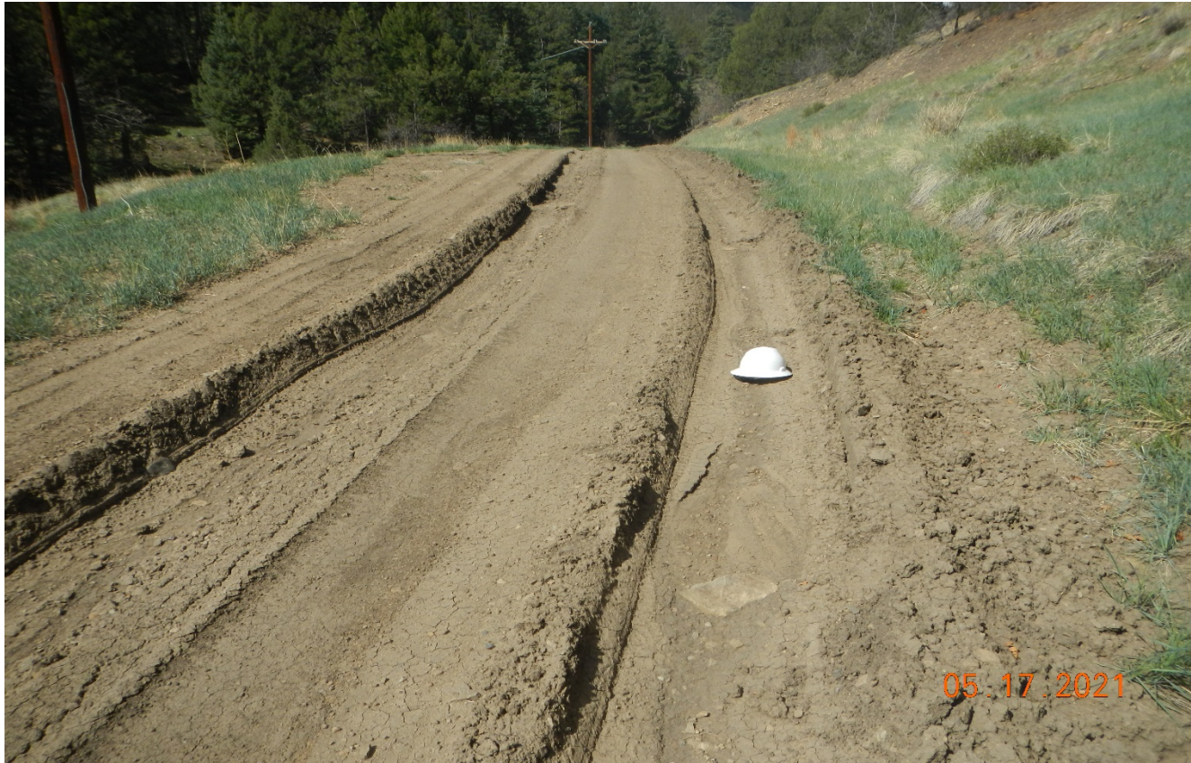
Photo 4. There is vehicle rutting along the main road. Areas of rutting need to be stabilized. Previous corrective action was not performed.
