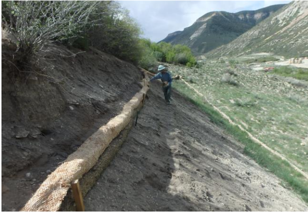
Double Stacking Wattle on CC 629-23-42 Pad
