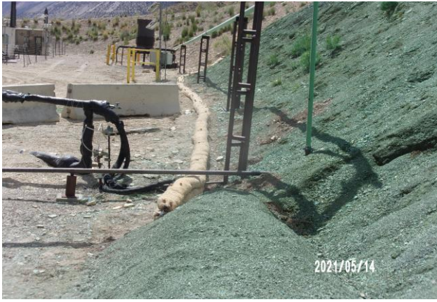
Wattle Installed below Cut-Slope and Piping
