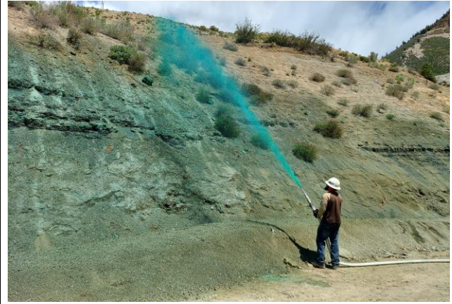
Treating Cut-Slope above New Containment Berm
