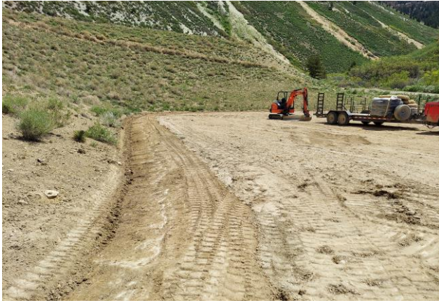
Containment Trench Installed on CC 797-03B Pad
