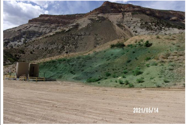
Cut-Slope Treated with Liquid Amenities and Nutrients
