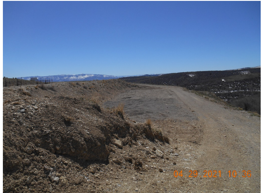
Generator housing, pump housing and tank battery removed.
