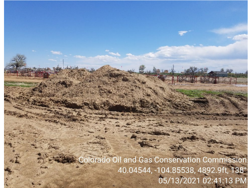
Photo 4 – Soil stored on location with inadequate BMPs.
