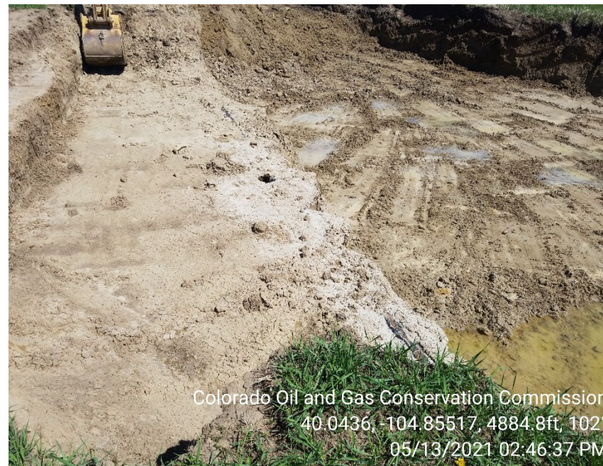
Photo 4 – Exposed flowline in open excavation.
