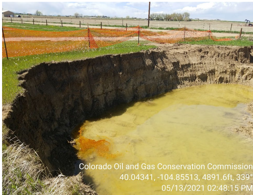
Photo 3 – Spill excavation. Impacts appear to remain in situ. Hydrocarbons observed on groundwater in open excavation.
