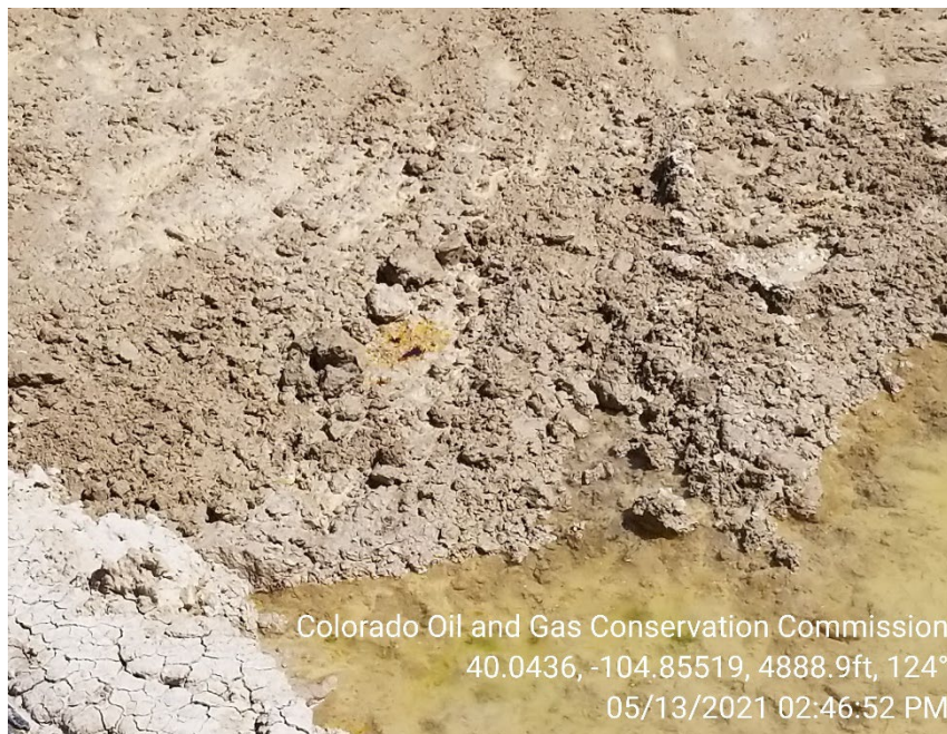
Photo 5 – Spill excavation. Impacts appear to remain in situ. Hydrocarbons observed on groundwater in open excavation.
