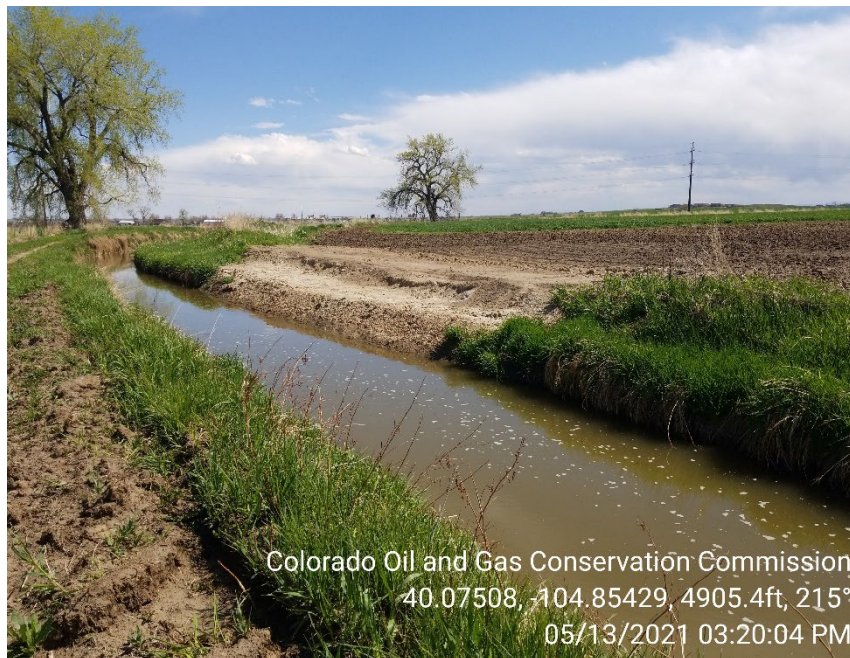
Photo 1 – Spill area. Excavation has been backfilled disturbed surfaces have been ripped. Canal is now active.
