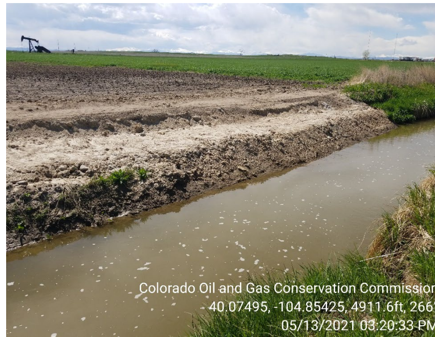
Photo 2 – Rebuilt ditch wall
