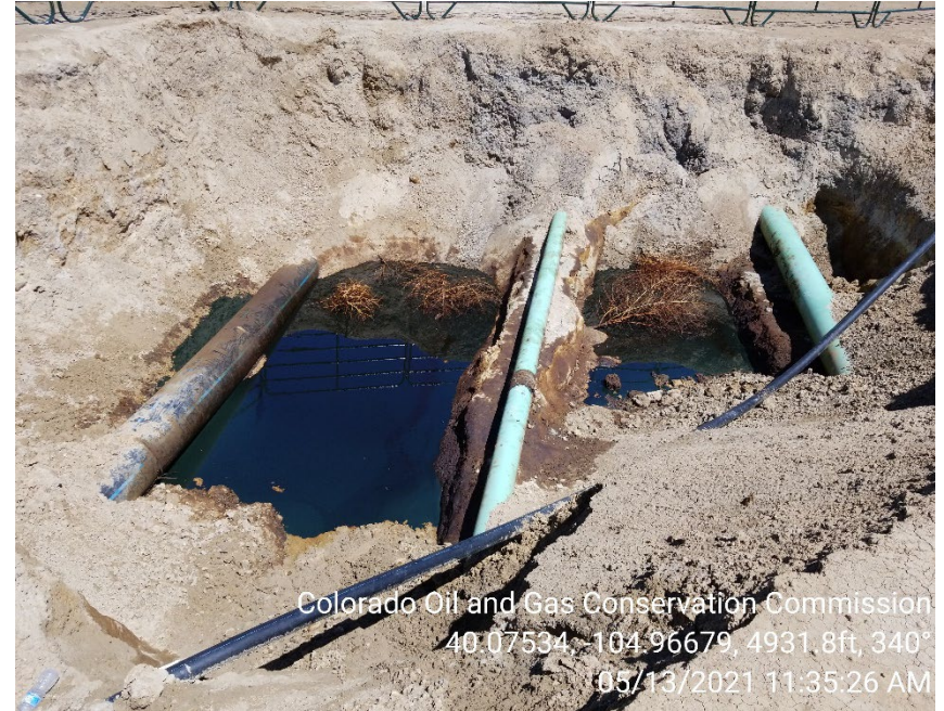
Photo 2 – Open excavation. Free product observed on groundwater. Impacts remain in situ.
