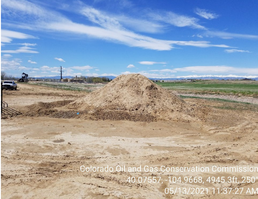
Photo 3 – Soils stored on location with inadequate BMPs
