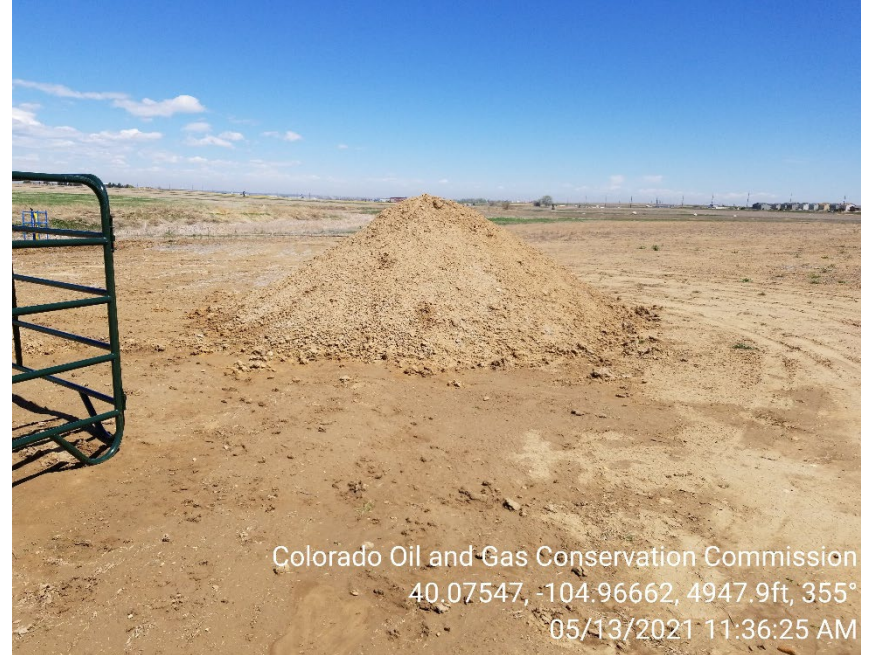
Photo 4 – Soils stored on location with inadequate BMPs
