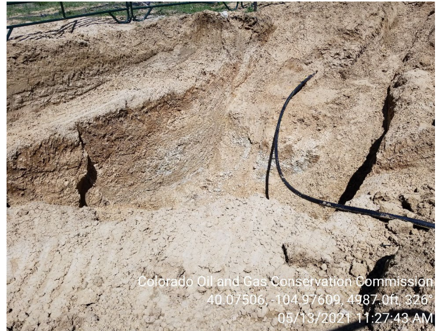
Photo 2 – Spill excavation.
