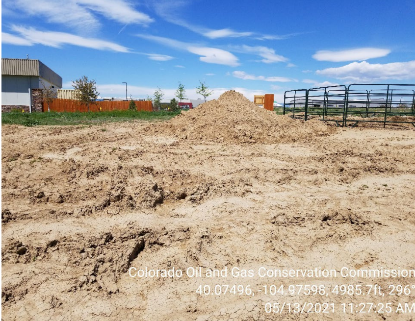
Photo 5 – Soils stockpiled on location with inadequate BMPs.
