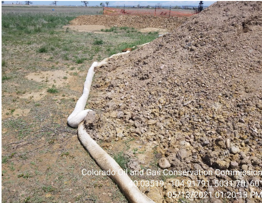
Photo 7 – Soils stored on location with inadequate BMPs
