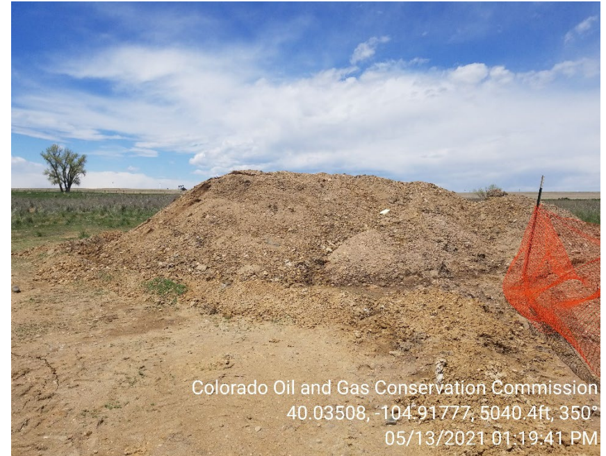
Photo 8 – Soils stored on location with inadequate BMPs
