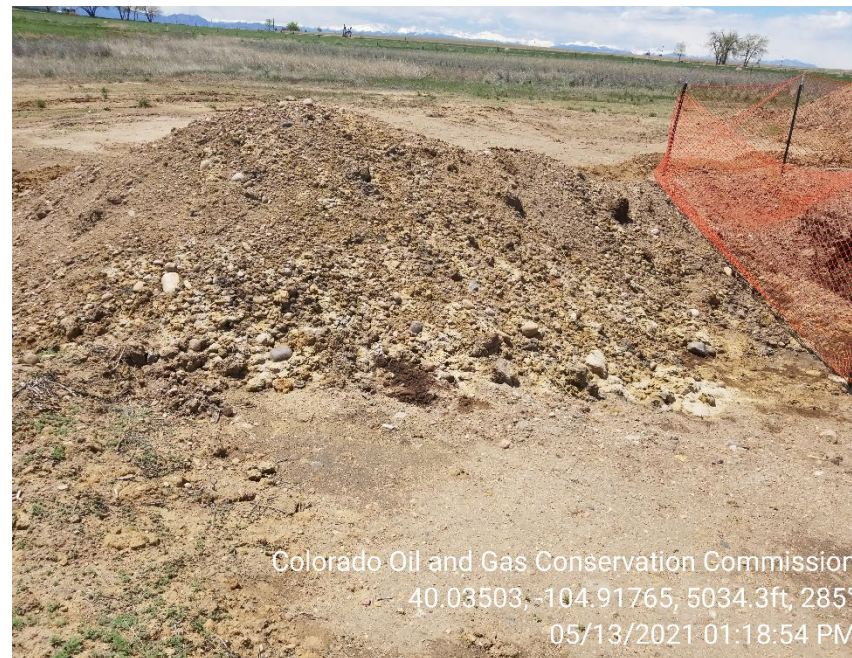
Photo 10 – Soils stored on location with inadequate BMPs
