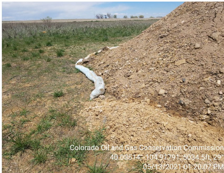
Photo 9 – Soils stored on location with inadequate BMPs
