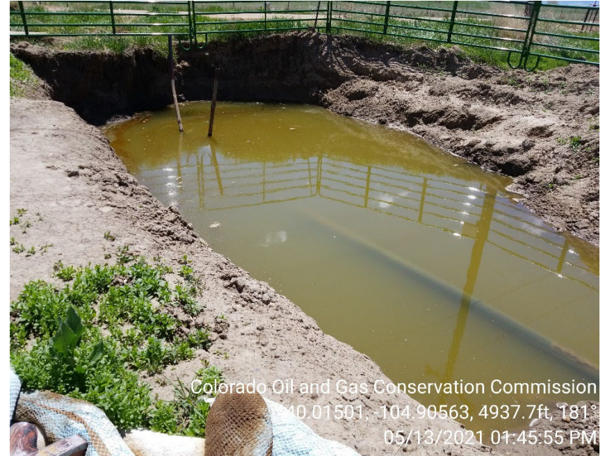
Photo 4 – Open excavation. Impacts appear to remain in situ. Hydrocarbons observed on groundwater.
