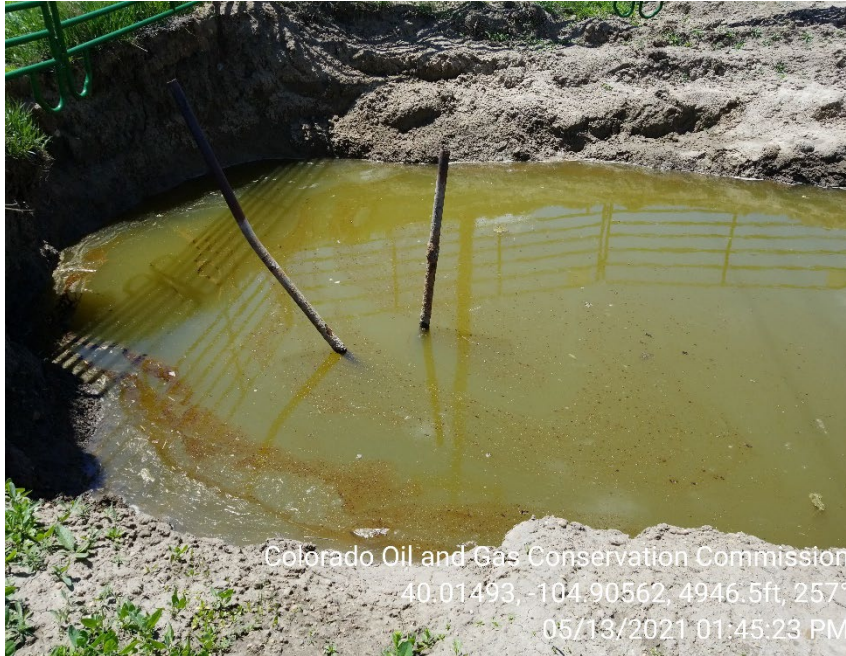
Photo 3 – Open excavation. Impacts appear to remain in situ. Hydrocarbons observed on groundwater.
