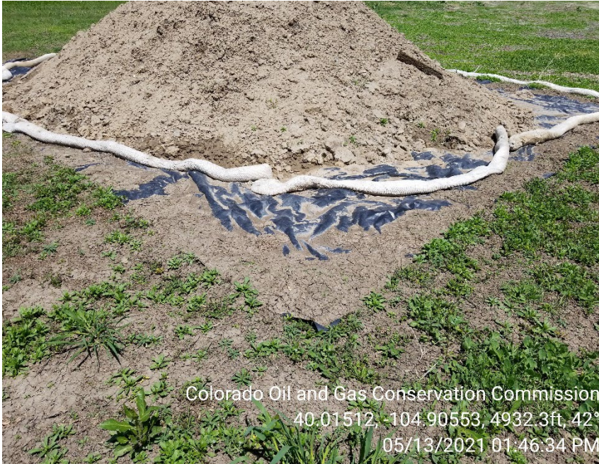
Photo 5 – Soil stored on location. Lining present under soil stockpile but BMPs are inadequate to prevent stormwater runoff.
