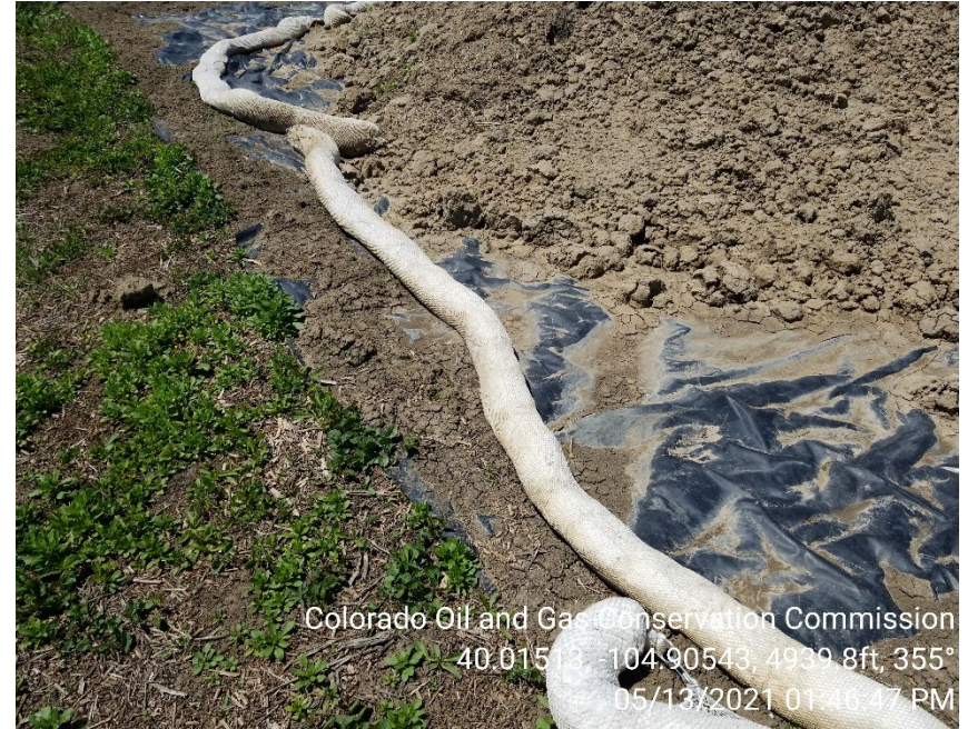
Photo 6 – Soil stored on location. Lining present under soil stockpile but BMPs are inadequate to prevent stormwater runoff.
