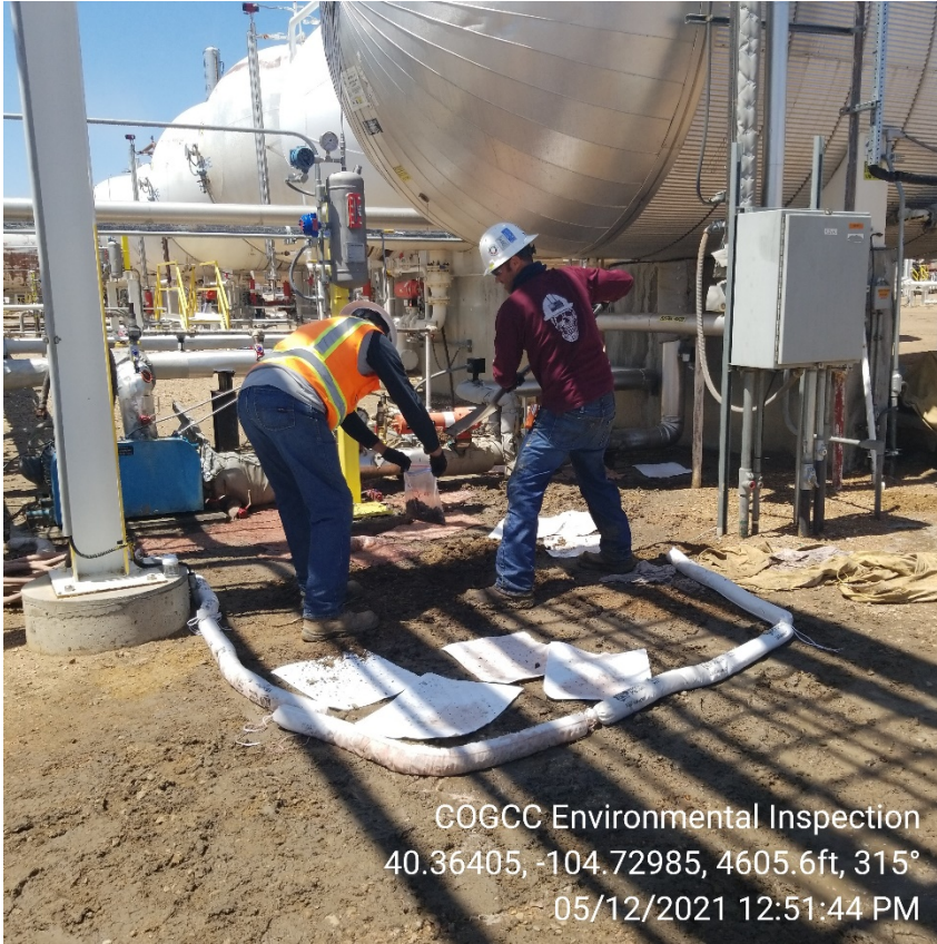
Photo 1 – Release source area: A ½” nipple valve broke, releasing condensate from a loading pump. Condensate mixed with rain water and spread across location.
