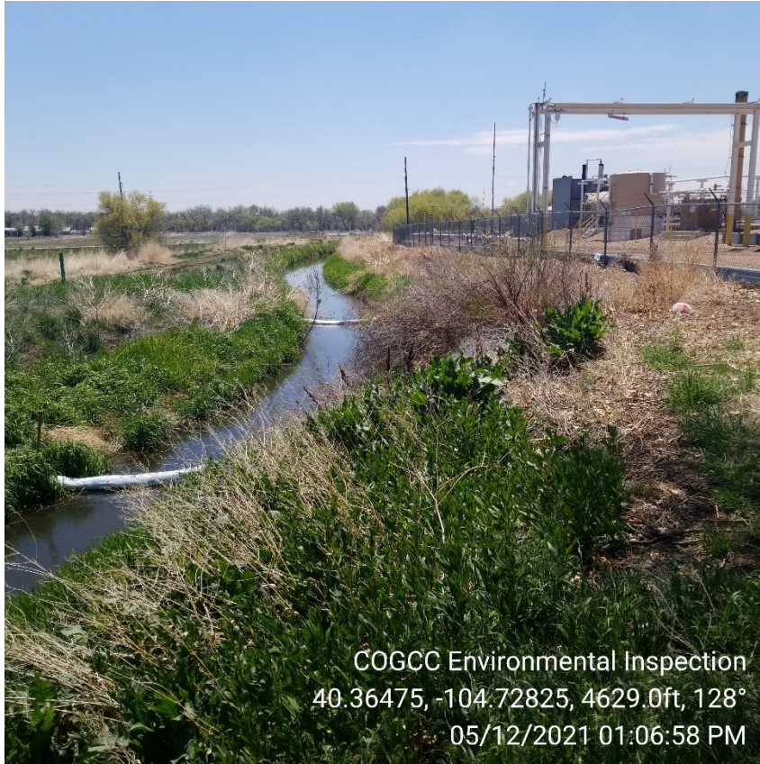
Photo 13 – Additional booms deployed down downstream of spill.
