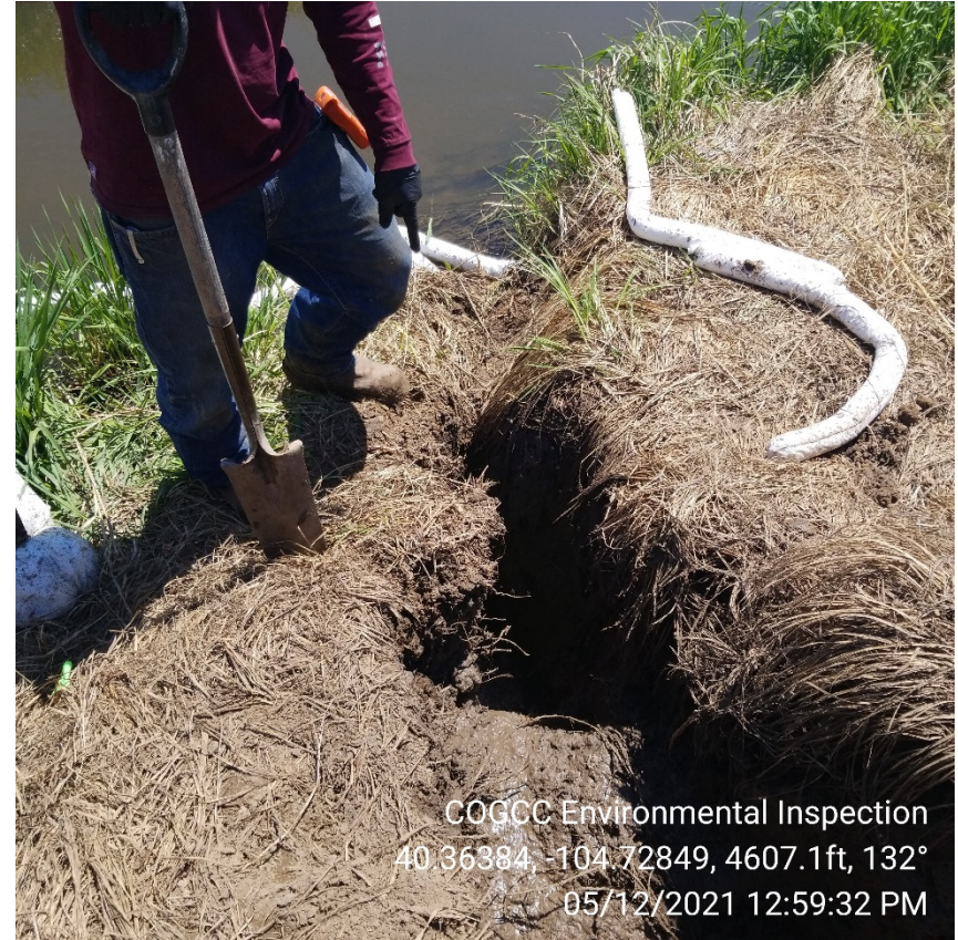
Photo 10 – Soil impact cleanup at eastern terminus of spill. Canal and booms in background.
