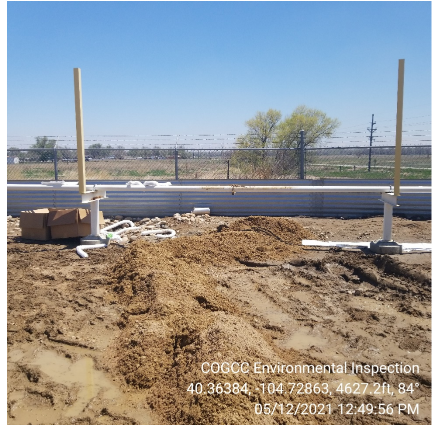
Photo 4 – Eastern terminus of the release. Impacts seeped under perimeter spill controls.
