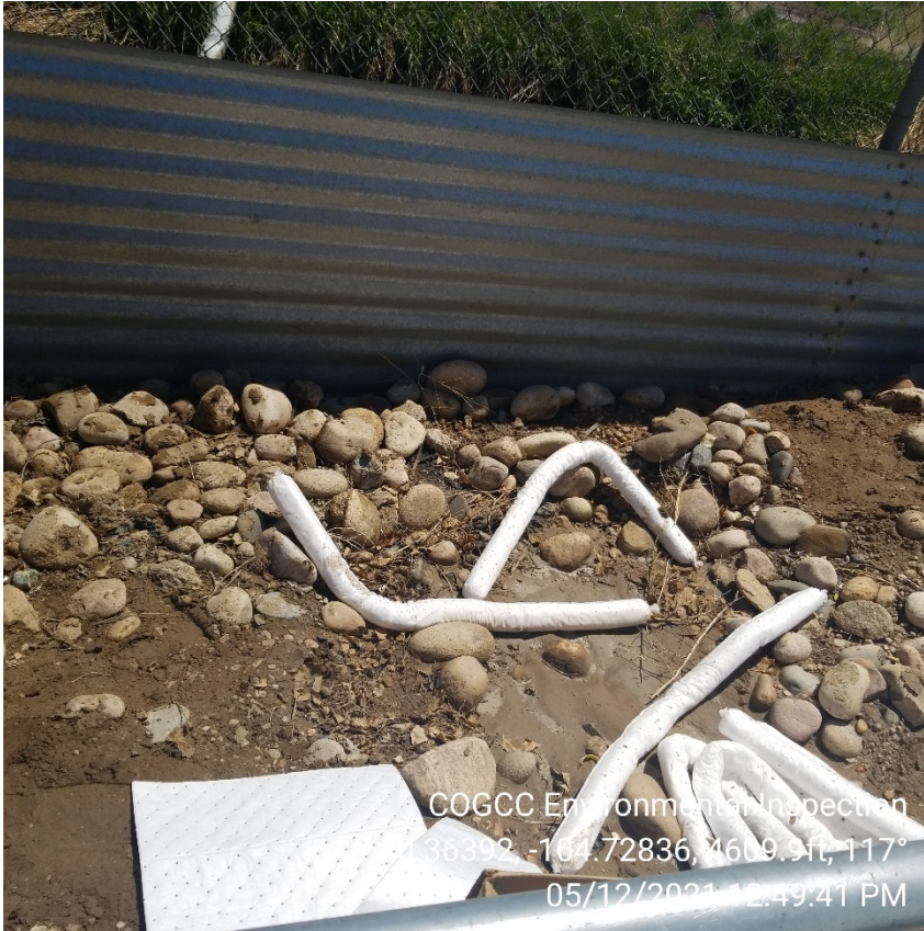
Photo 5 – Eastern terminus of the release. Impacts seeped under perimeter spill controls.
