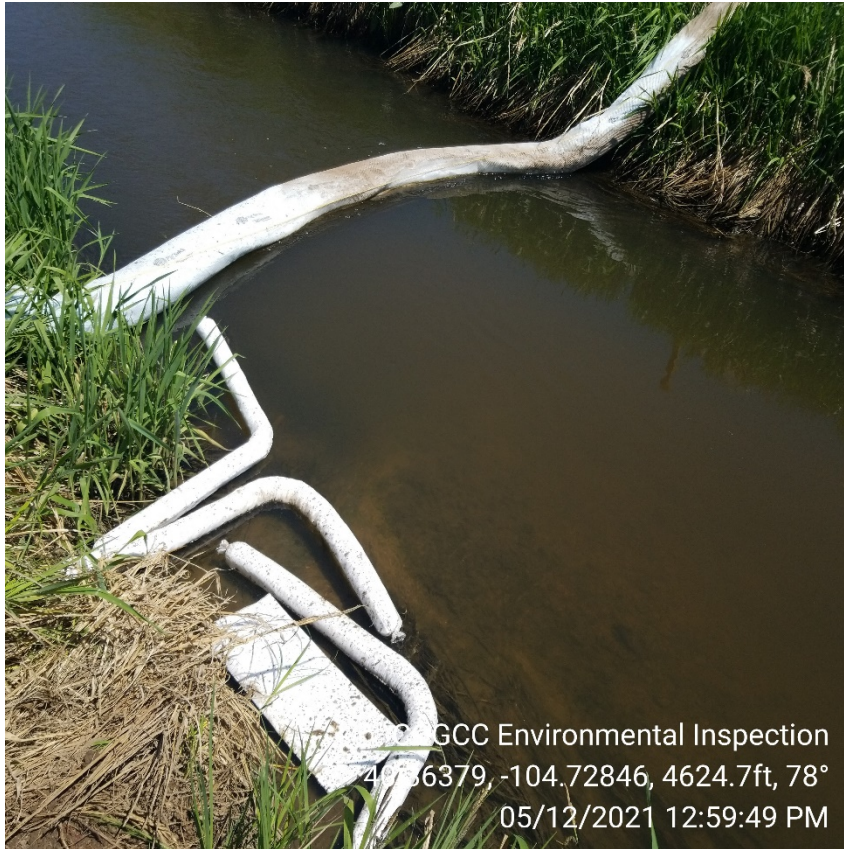
Photo 11 – Booms deployed in irrigation ditch to control hydrocarbons
