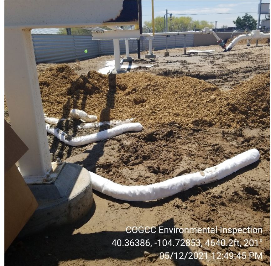
Photo 6 – Southeastern terminus of the release. Impacts seeped under perimeter spill controls.
