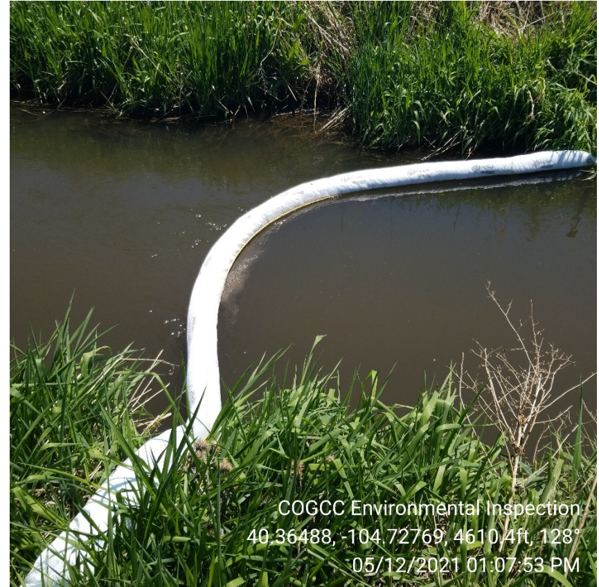
Photo 14 – Boom immediately down gradient of release area.
