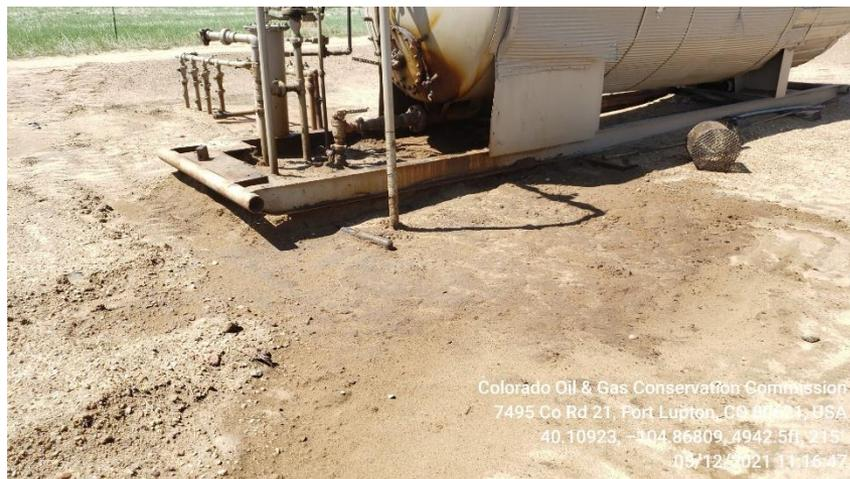
**Photo 9 stained soil around Horiz. Heated Sep.**
