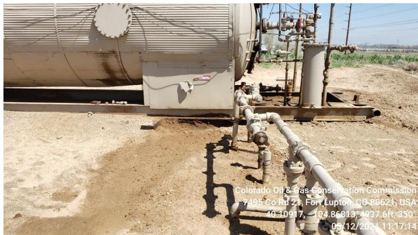
**Photo11 stained soil around Horiz. Heated Sep.**
