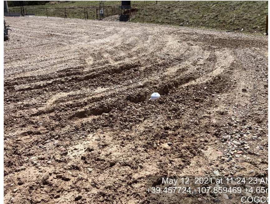
Lack of stabilization/compaction
