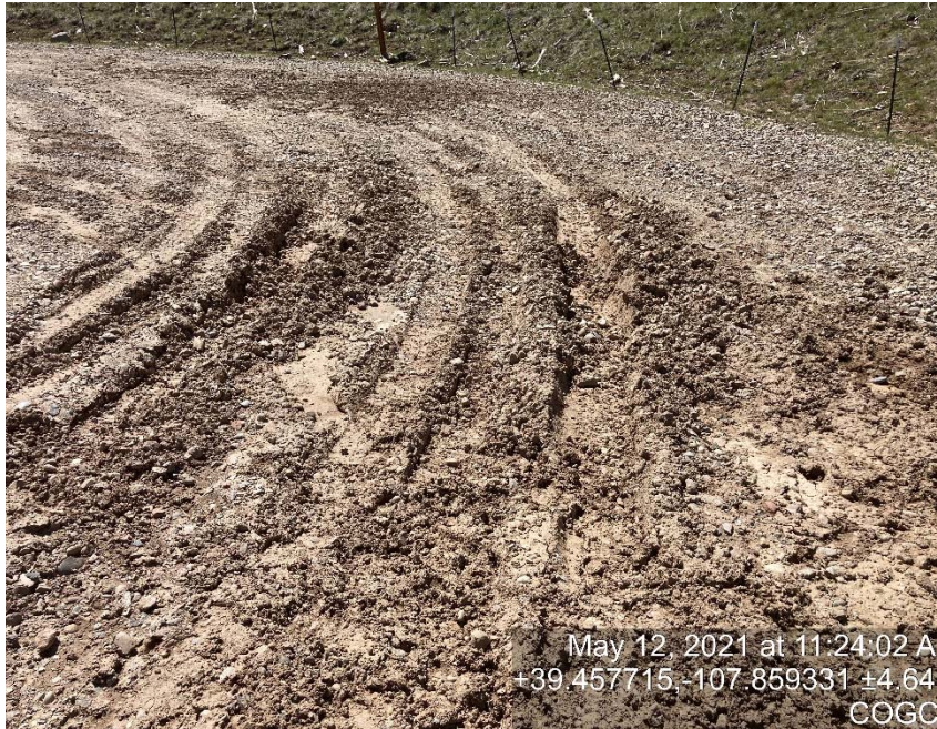
Lack of stabilization/compaction
