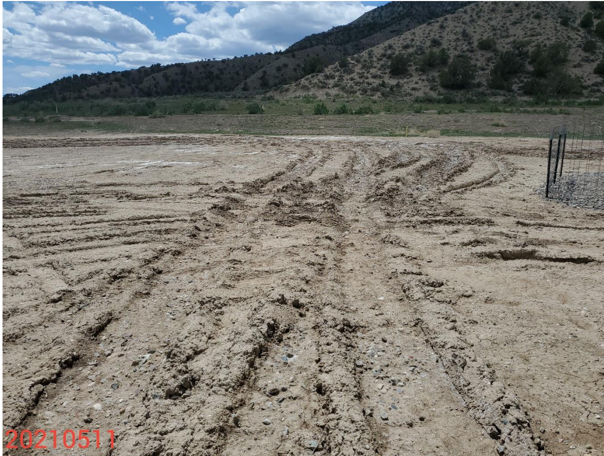
Photo 5 Photos 5-8 taken from the production area. Photos show control measures to stabilize and protect unpaved areas of the Location are missing or insufficient.
