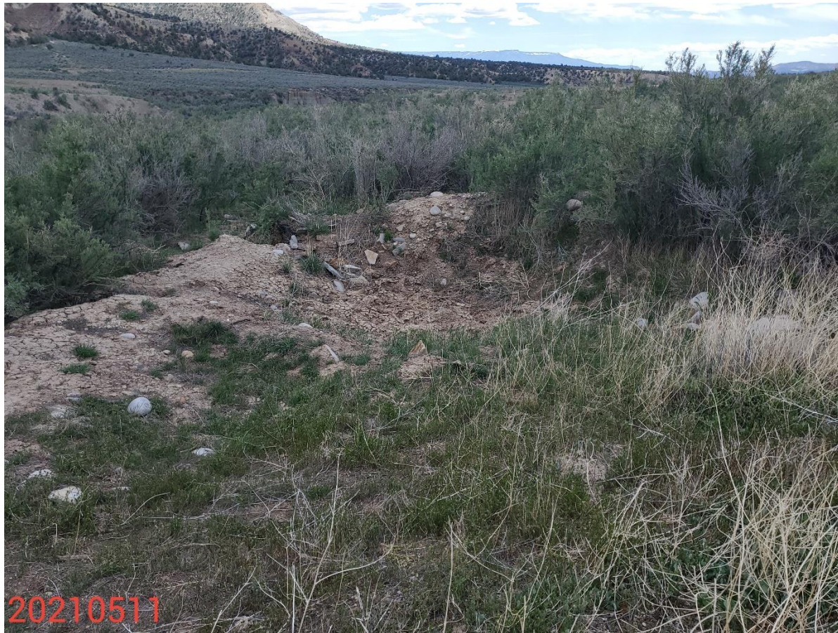
Photo 9: Photo taken from the sediment trap on the south end of the Location. Sediment trap has not been maintained in proper functioning condition.
