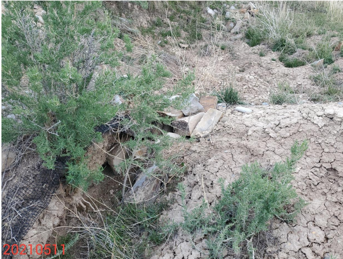
Photo 12: Photo taken from the sediment trap on the south end of the Location. Sediment trap has not been maintained in proper functioning condition. Erosion degradation evident.
