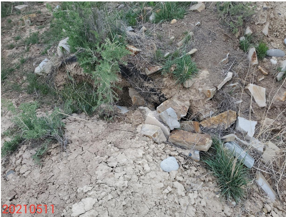
Photo 11: Photo taken from the sediment trap on the south end of the Location. Sediment trap has not been maintained in proper functioning condition. Erosion degradation evident. .
