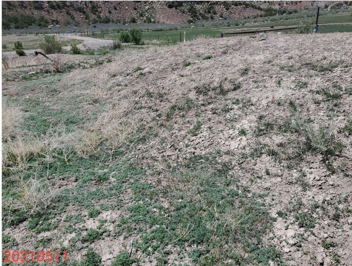
Photo 16: Photo taken from the soil stockpile on the northwest end of the Location. Photo shows vegetation observed on stockpile are undesirable weedy plant species. Stockpile not protected in accordance with Rule 1002.c
