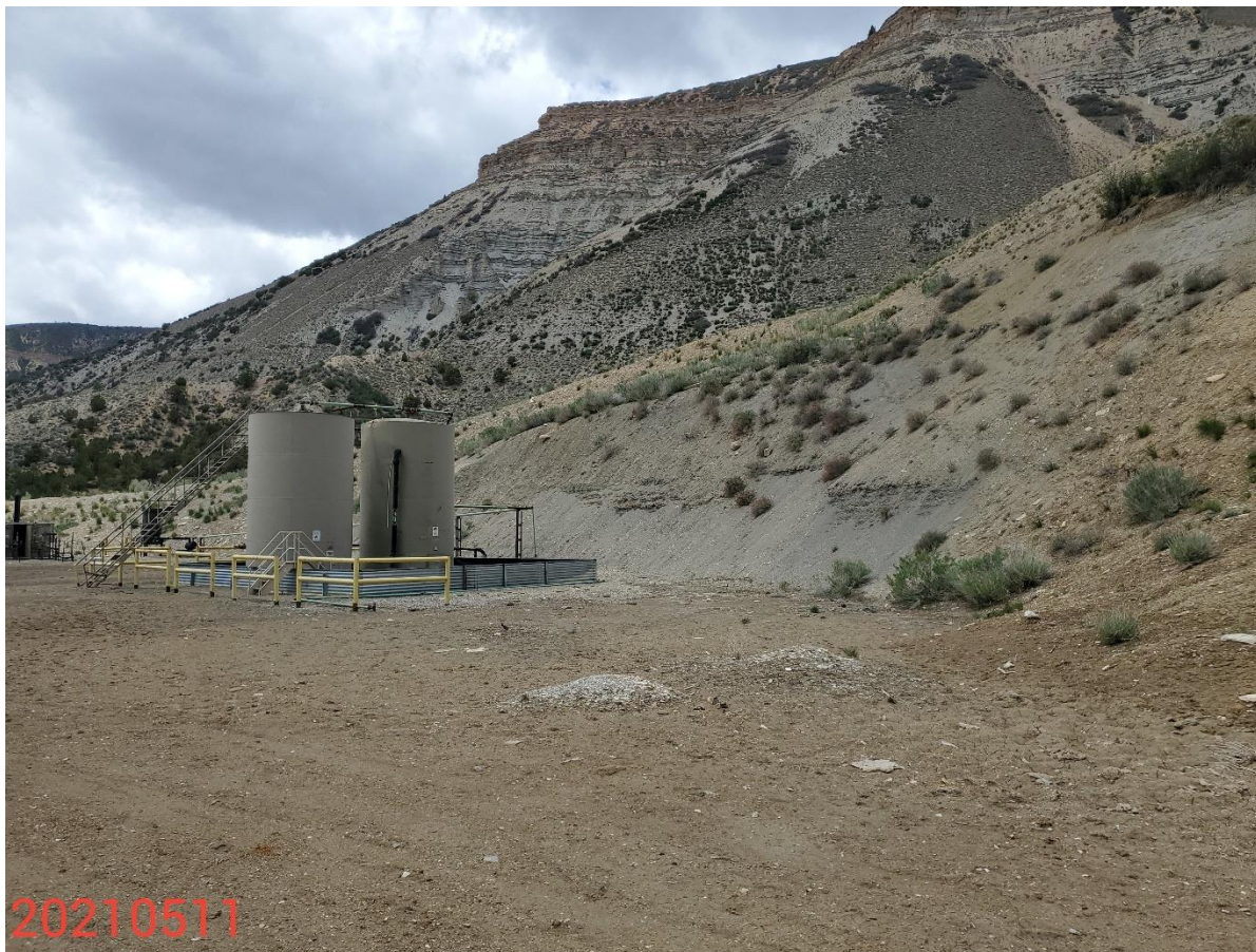
Photo 1: Photo taken from the production area, facing northwest. Photo shows cut slopes of the Location. Slopes/soils exposed; control measures to protect/stabilize slopes missing or insufficient.
