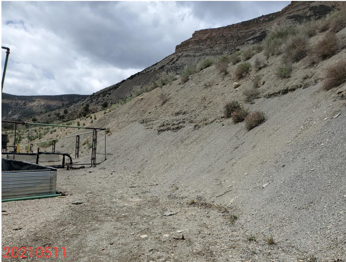
Photo 2: Photo taken from the north end of the Location, facing west. Photo shows soils at cut slope are exposed; control measures to protect/stabilize slopes missing or insufficient.
