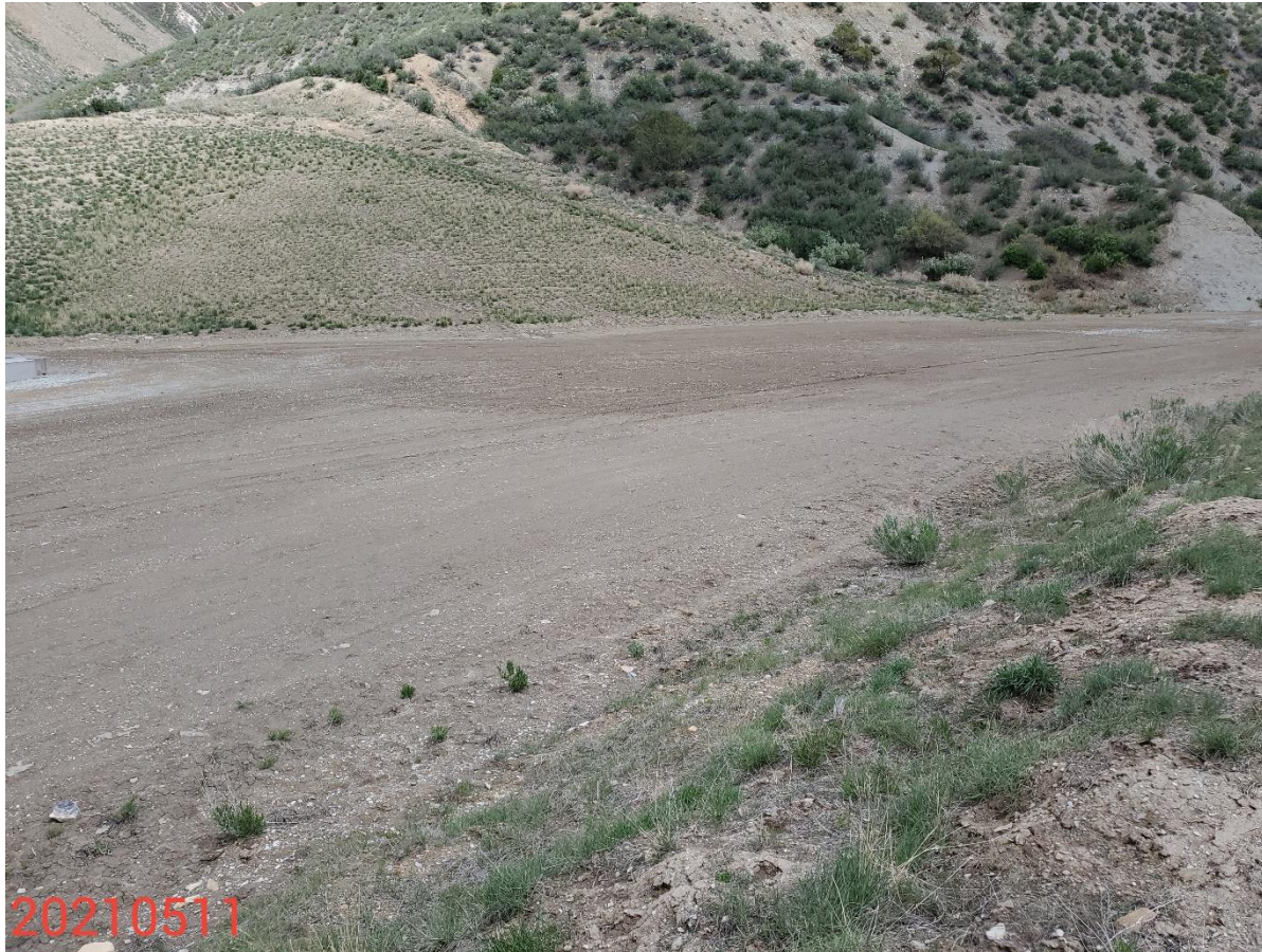
Photo 6: Photo taken from the slopes on the west end of the Location. Photo shows erosion degradation remains evident on the slopes; control measures to stabilize/protect slopes remain missing or insufficient.
