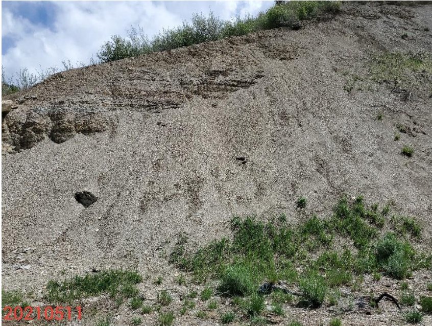
Photo 7: Photo taken from the cut slopes on the west end of the Location. BMPs to provide long term protection and stabilization are missing or insufficient.
