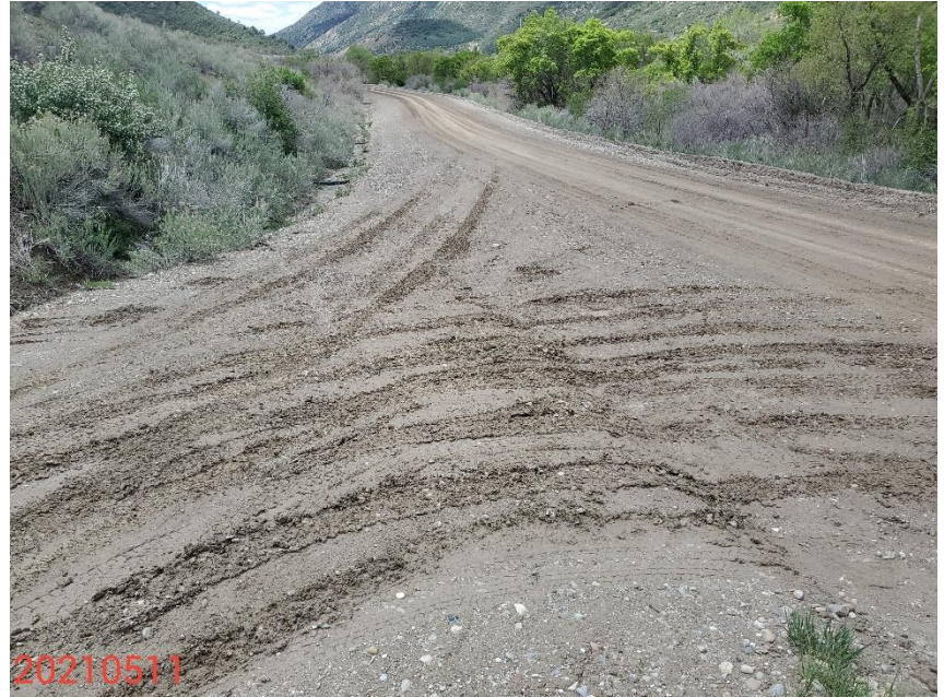
Photo 10: Photo taken from the access road entrances, facing southwest. Photo shows BMPs to stabilize production areas/access road and to prevent off-location sediment transport during wet conditions are missing or insufficient
