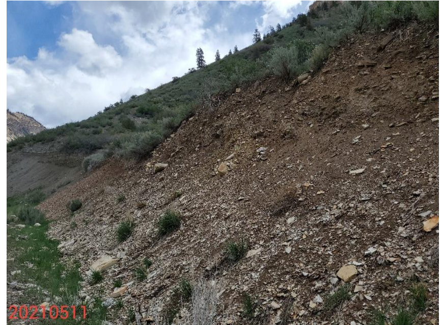
Photo 8: Photo taken from the cut slopes on the west end of the Location. BMPs to provide long term protection and stabilization are missing or insufficient.
