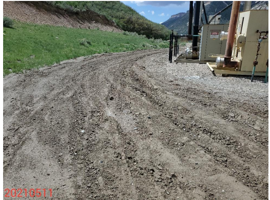
Photo 6: Photo taken from the tank battery. Photo shows control measures to stabilize the production area are missing or insufficient.
