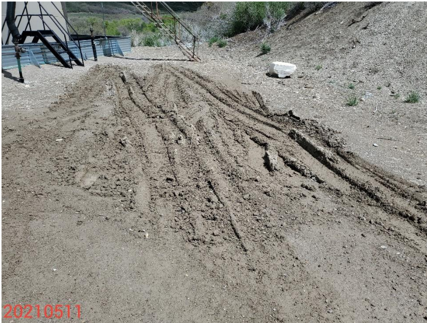
Photo 5: Photo taken from the tank battery. Photo shows control measures to stabilize the production area are missing or insufficient.
