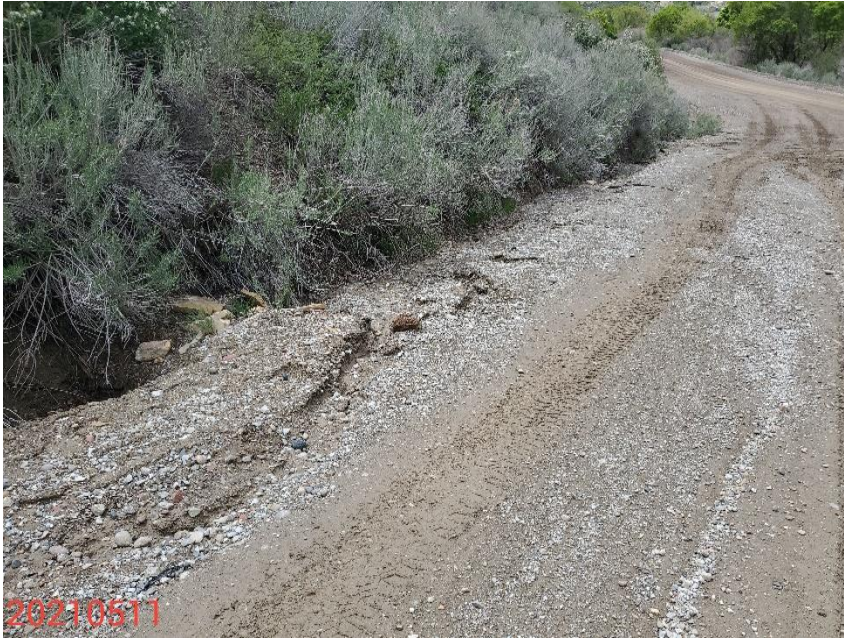
Photo 9: Photo taken from the access road. Photo shows erosion degradation along access road.
