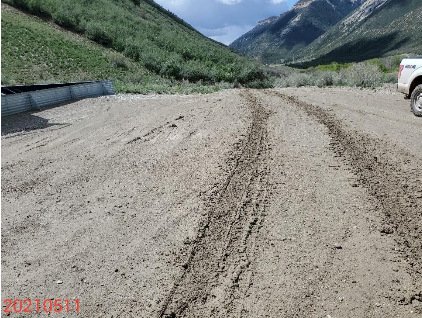
Photo 11: Photo taken from the southwest end of the Location, facing south. Photo shows control measures to stabilize the production area are missing or insufficient.
