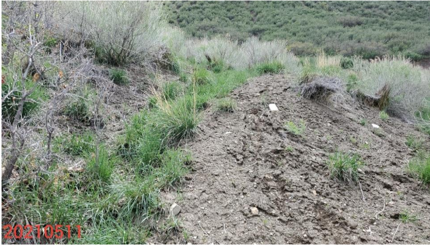
Photo 9: Photo taken from the stormwater ditch/berm on the northwest end of the Location. Photo shows areas where erosion was observed on the berm.
