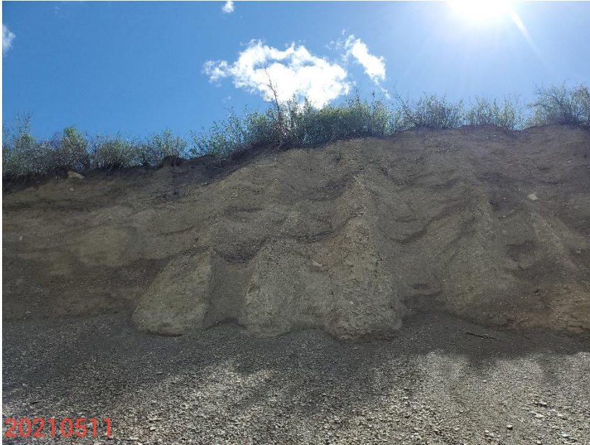
Photo 5: Photo taken from the cut slopes on the west end of the Location. BMPs to provide long term protection and stabilization are missing or insufficient.
