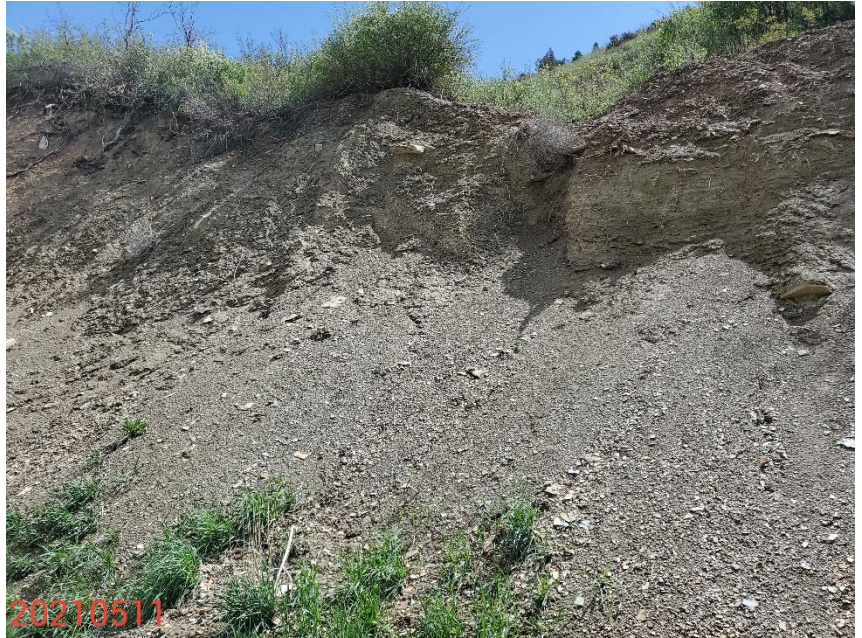
Photo 6: Photo taken from the cut slopes on the west end of the Location. BMPs to provide long term protection and stabilization are missing or insufficient.
