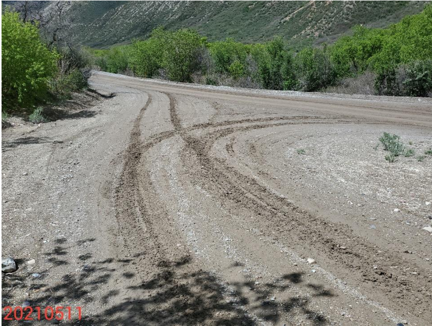
Photo 13: Photo taken from the access road entrances, facing southwest. Photo shows BMPs to stabilize production areas/access road and to prevent off-location sediment transport during wet conditions are missing or insufficient
