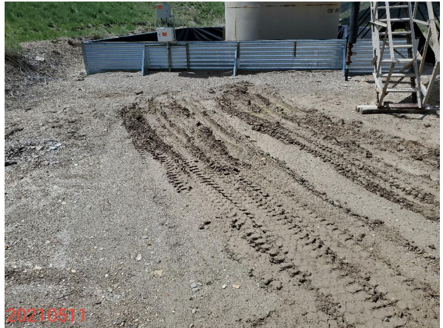
Photo 10: Photo taken from the tank battery. Photo shows control measures to stabilize the production area are missing or insufficient.
