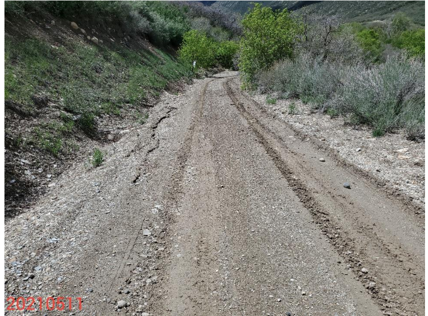
Photo 12: Photo taken from the access road, facing south. Photo shows example of erosion degradation observed on access road.
