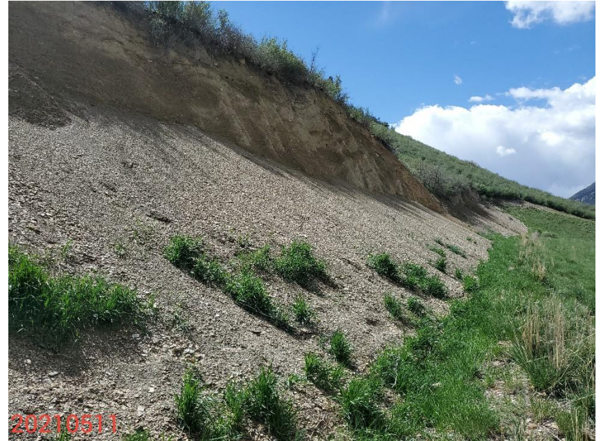
Photo 4: Photo taken from the cut slopes on the west end of the Location. Slopes have not revegetated; BMPs to provide long term protection and stabilization are missing or insufficient.
