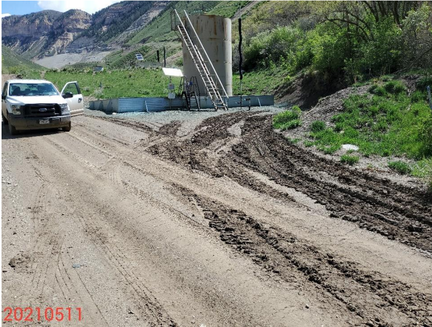
Photo 5: Photo taken from the access road, southwest of the tank, facing northeast. Photo shows control measures to stabilize the production areas/access road and to prevent off-location sediment transport during wet conditions have not been maintained in proper functioning condition.
