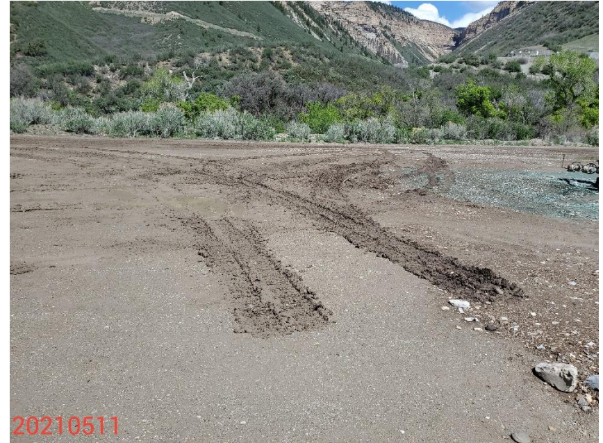
Photo 2: Photo taken from the production area, facing northwest. Photo shows control measures to stabilize the production areas/access road and to prevent off-location sediment transport during wet conditions have not been maintained in proper functioning condition.
