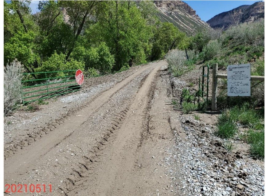
Photo 6: Photo taken from the access road entrance, facing north. Cattle guard has filled with sediment. Deep ruts observed along areas of access road.
