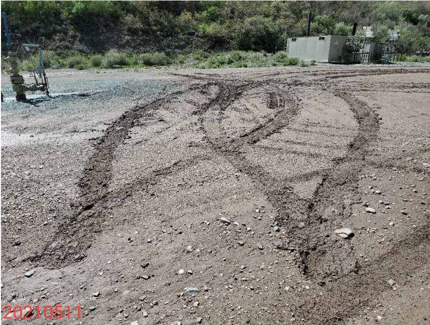
Photo 1: Photo taken from the production area, facing south. Photo shows control measures to stabilize the production areas/access road and to prevent off-location sediment transport during wet conditions have not been maintained in proper functioning condition.
