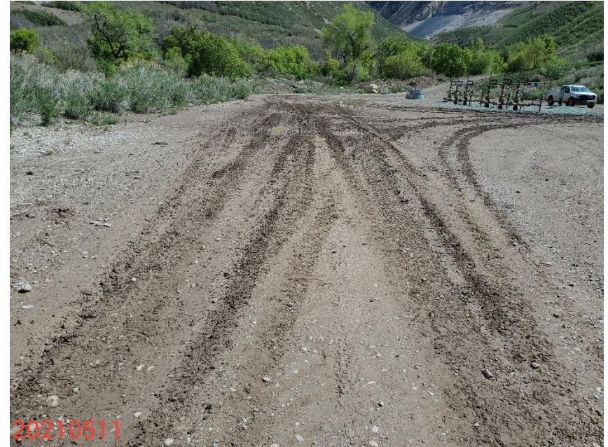
Photo 4: Photo taken from the southwest end of the production area, facing northeast. Photo shows control measures to stabilize the production areas/access road and to prevent off-location sediment transport during wet conditions have not been maintained in proper functioning condition.
