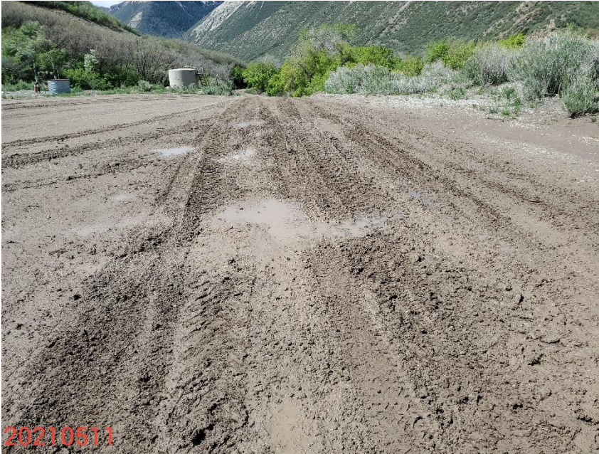
Photo 3: Photo taken from the west end of the production area, facing southwest. Photo shows control measures to stabilize the production areas/access road and to prevent off-location sediment transport during wet conditions have not been maintained in proper functioning condition.
