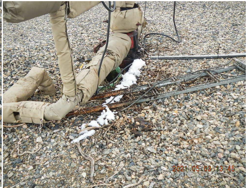
Oil staining, trash/debris near wellhead.
