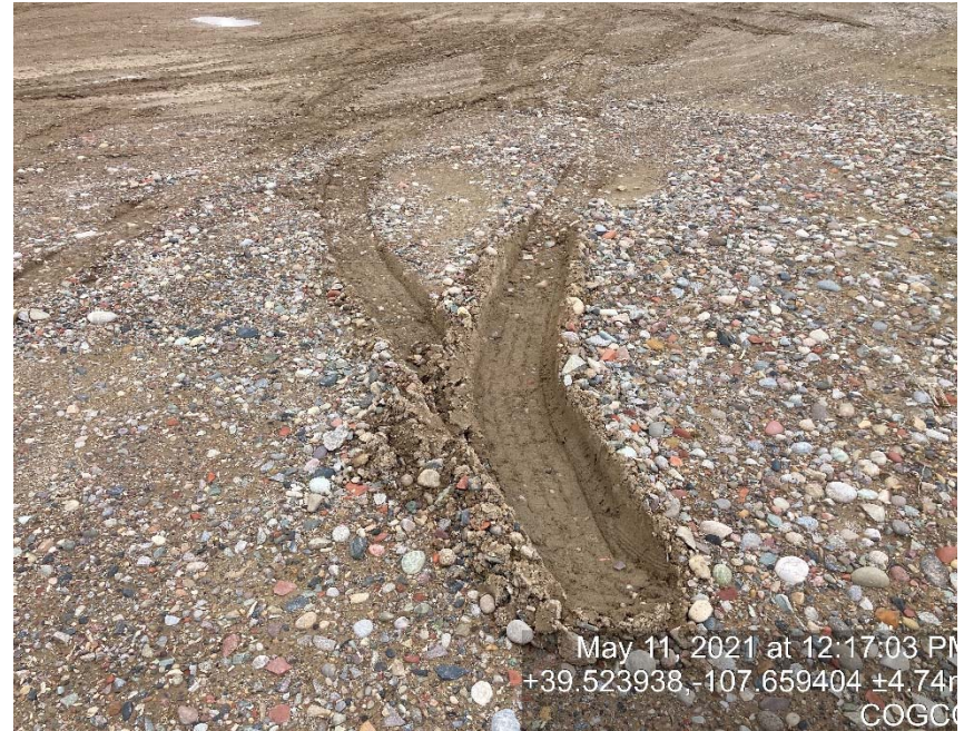
Lack of stabilization/compaction
