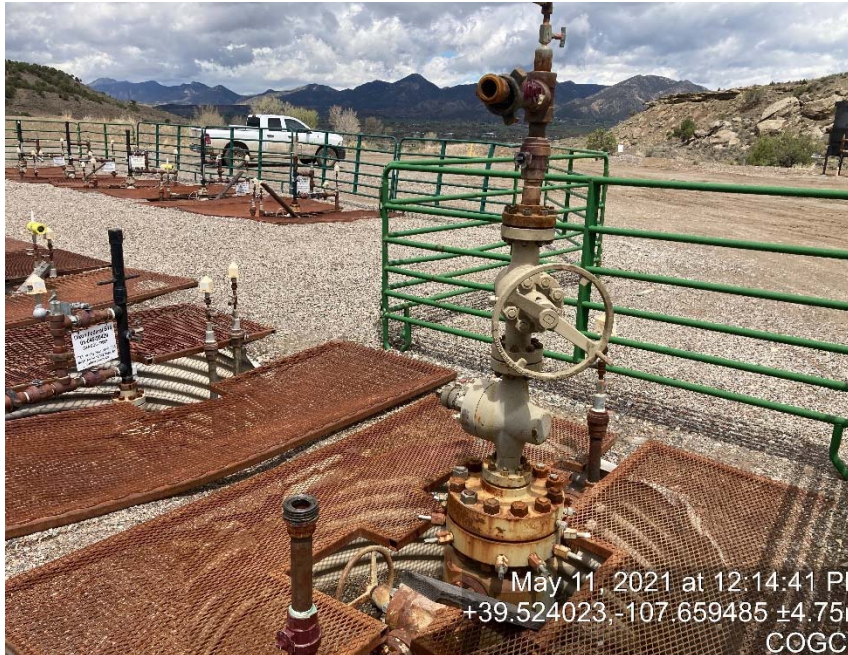
Location/ dismantled well head
