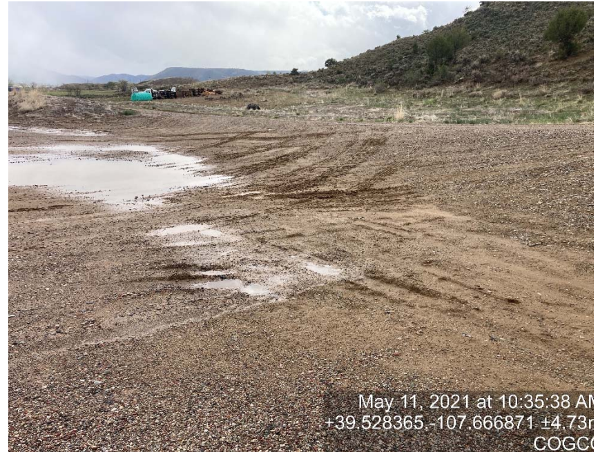
Lack of stabilization/compaction
