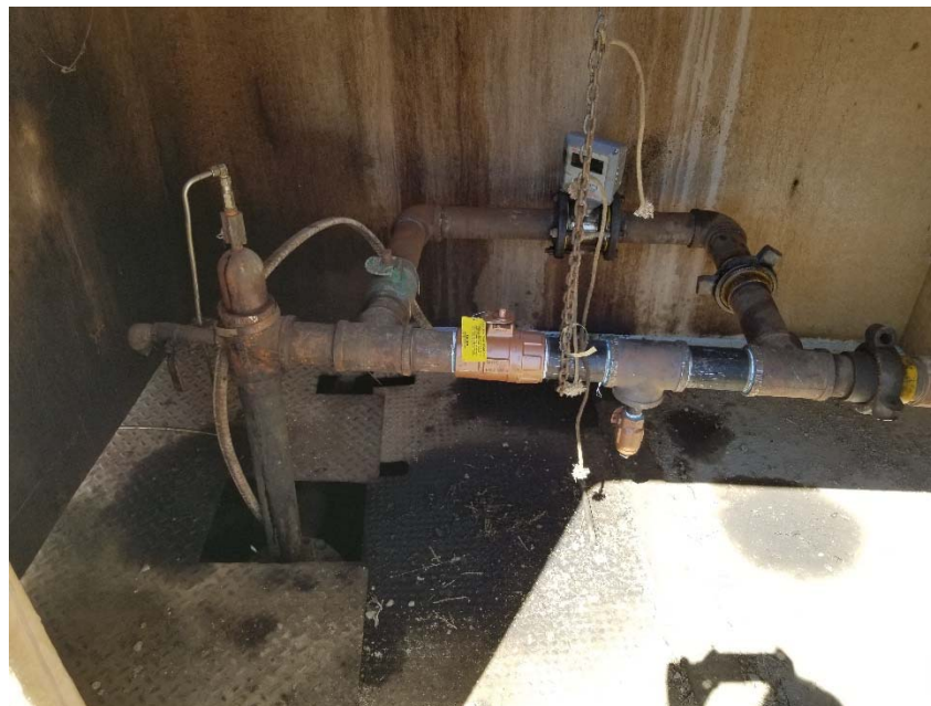
Photo 2. No bradenhead access apparent.
