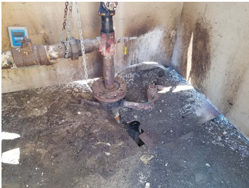
Photo 2. No bradenhead access apparent.
