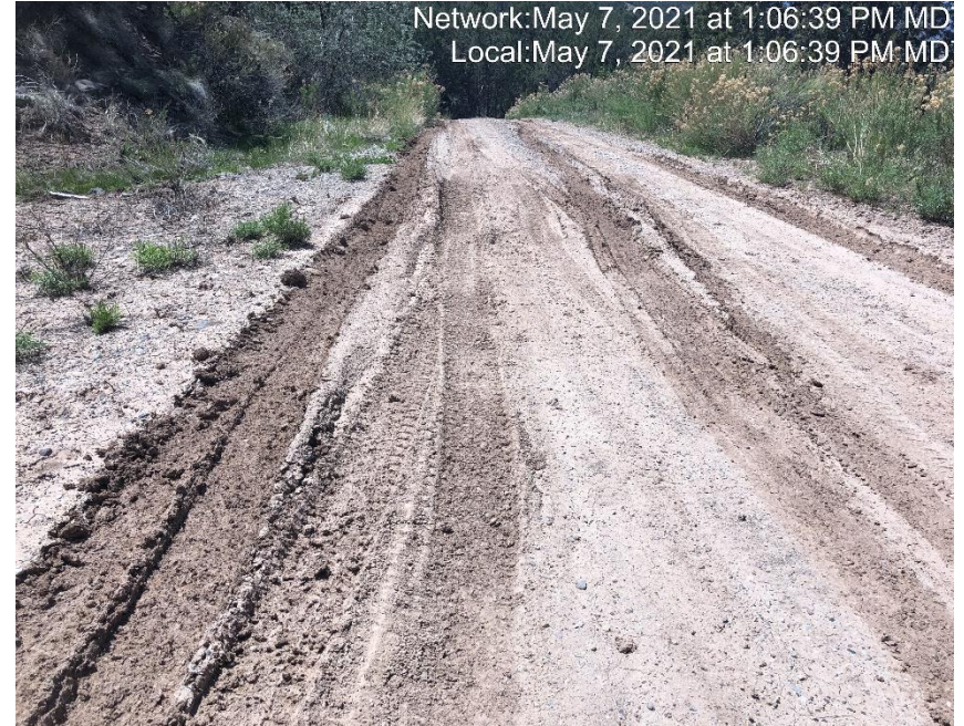
Photo #3759 No form of tracking BMP located at entrance to location.
