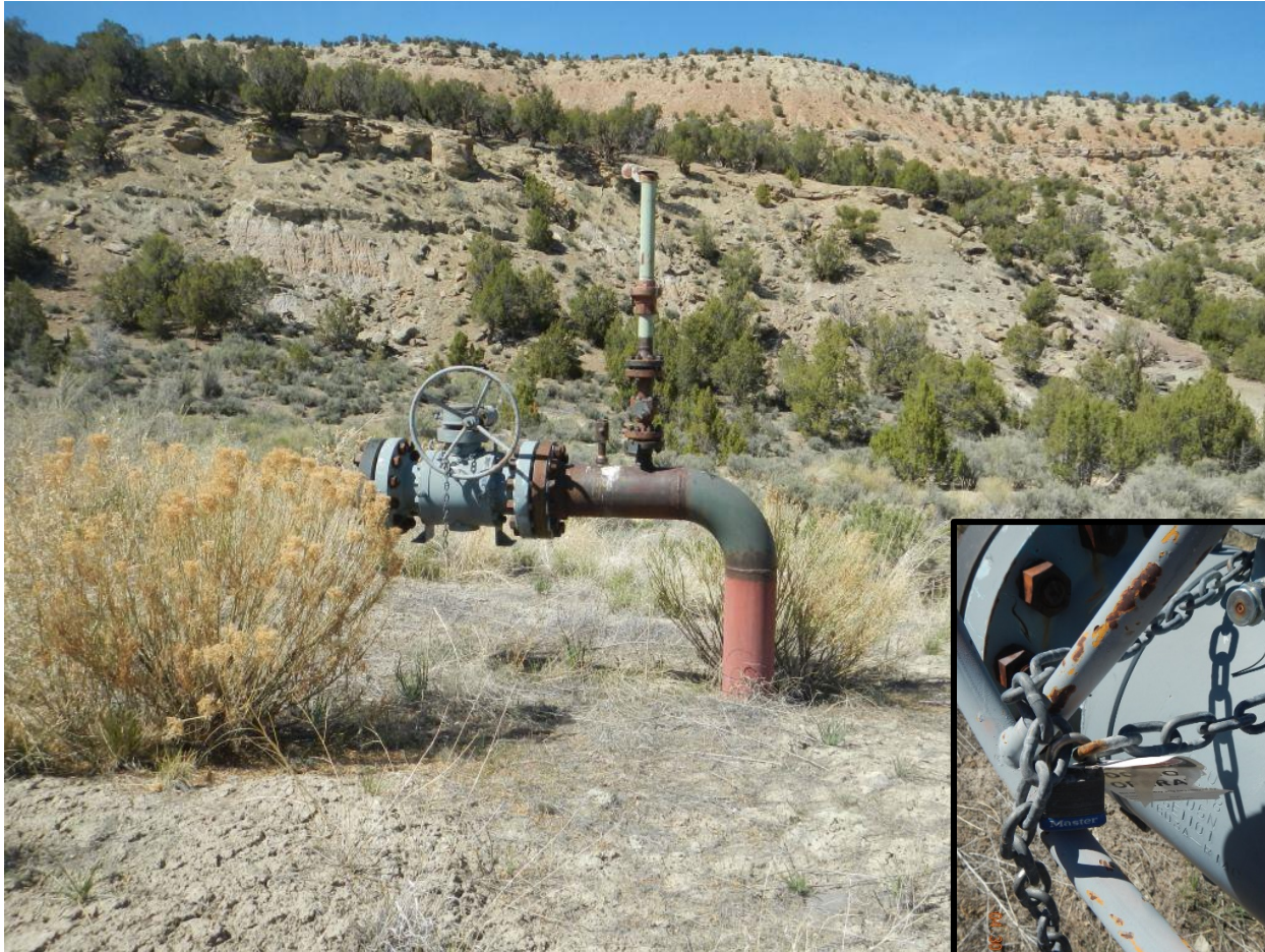
Photo#4: Riser, on North edge of Location; insert Handle Lockout, Tag out.
